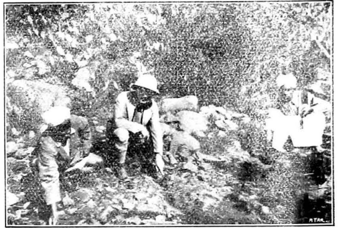
Fig. 32. — Mettur: Drainage of seepage water.
