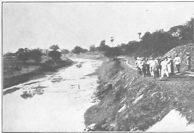
Fig. 7. — Murshidabad. — Attempt to restore a dead river by conducting silty water from the Ganges.
