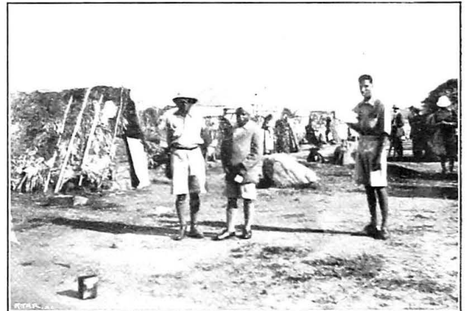
Fig. 34. — Mettur: Temporary coolie line.
