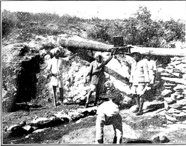
Fig. 31. — Mettur: Drip-can oiling of drains.
