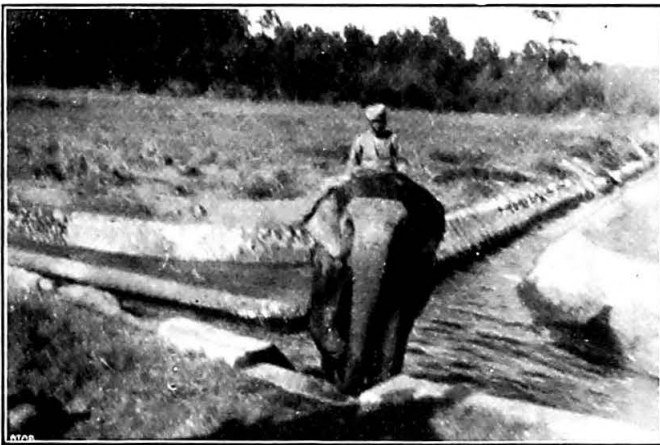
Fig. 28. — United Provinces: Drainage of the Sarda Canal. Bridge head at Banbassa.
