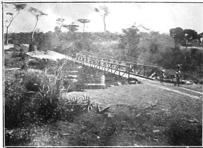
13. Bridge over the River Kibali.
