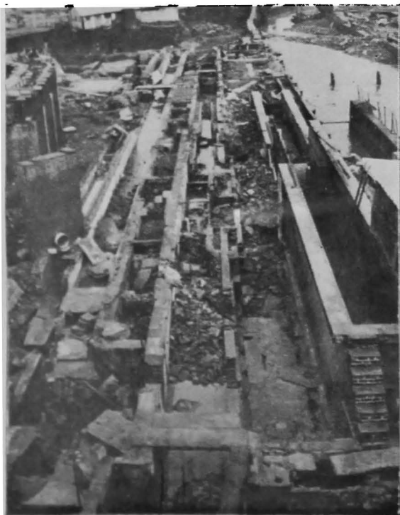
Damage to the Models after the Breach
