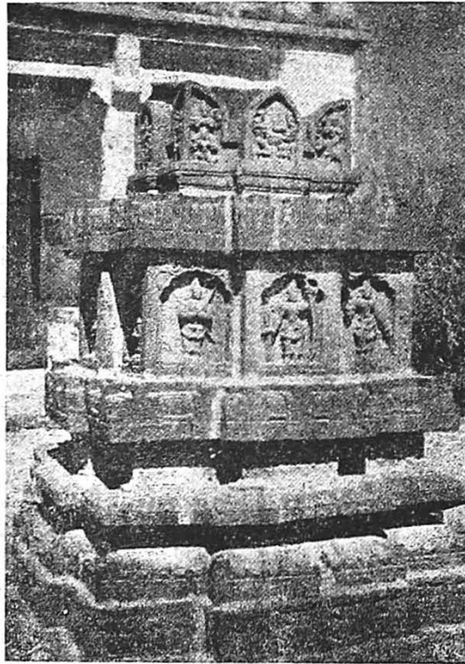
Fig. 3.— Structure for Tulasi, carved in trap, Ramallakota.
