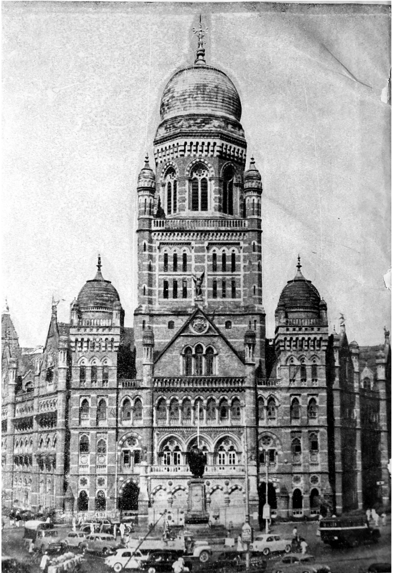
MUNICIPAL HEAD OFFICES
