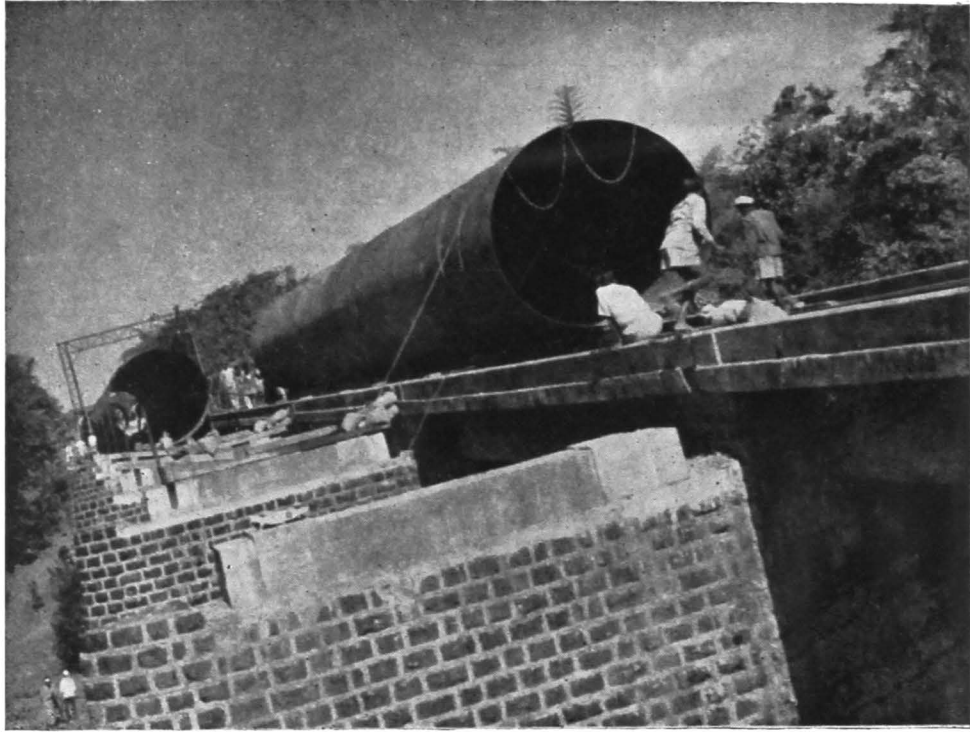
120" dia. Pipeline, 108 Ft. long ready to be rolled on Tansa Bridge
