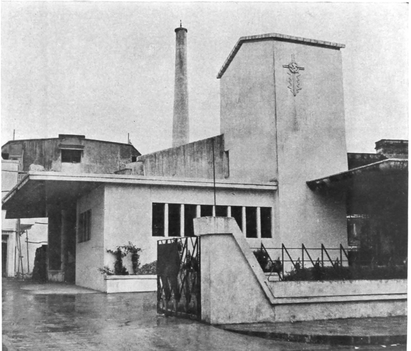
The new Electric Crematorium at Chandanwadi, first of its kind in India, affording such amenities as a reception room, rest rooms, a hall for performing religious rites and separate bath rooms for men and women.
