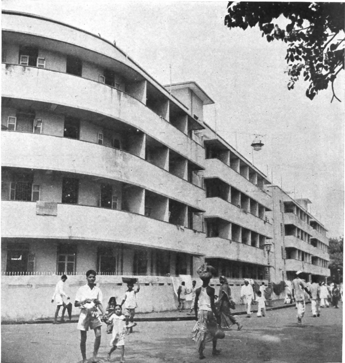
Housing for Conservancy Staff at Bapty Road Yard Front view of the buildings facing Bapty Road
