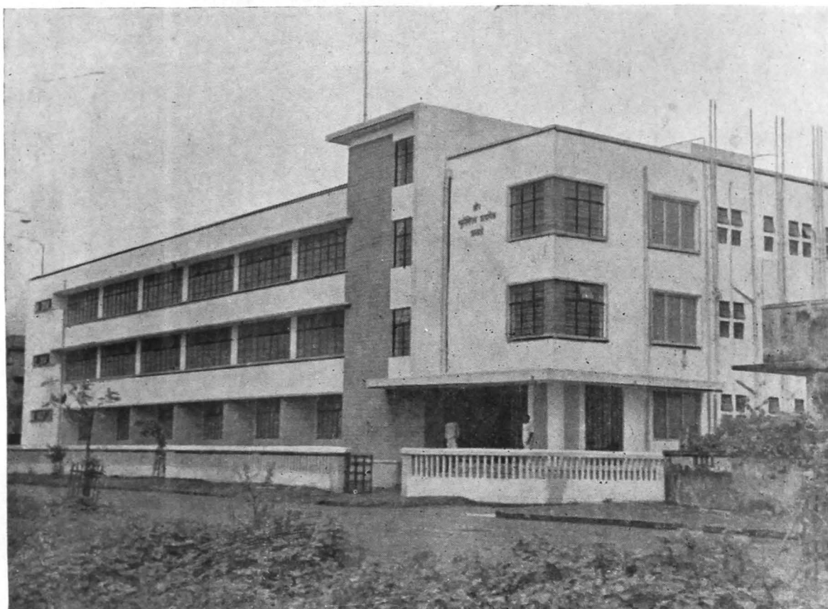
New School Building at Sion. The building consists of 31 class rooms. There is a covered playarea on ground floor for drills etc. during the monsoon and a big hall on first floor for various activities. An innovation is the provision of a number of plaster panels in bas-relief depicting animal life and geometrical figures and numerals etc.
