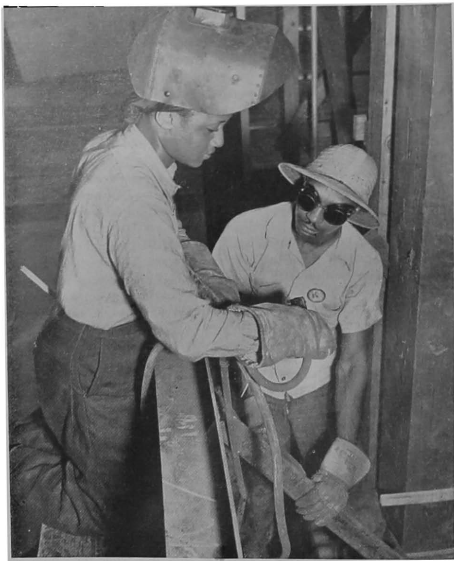
Welder in a shipyard.
