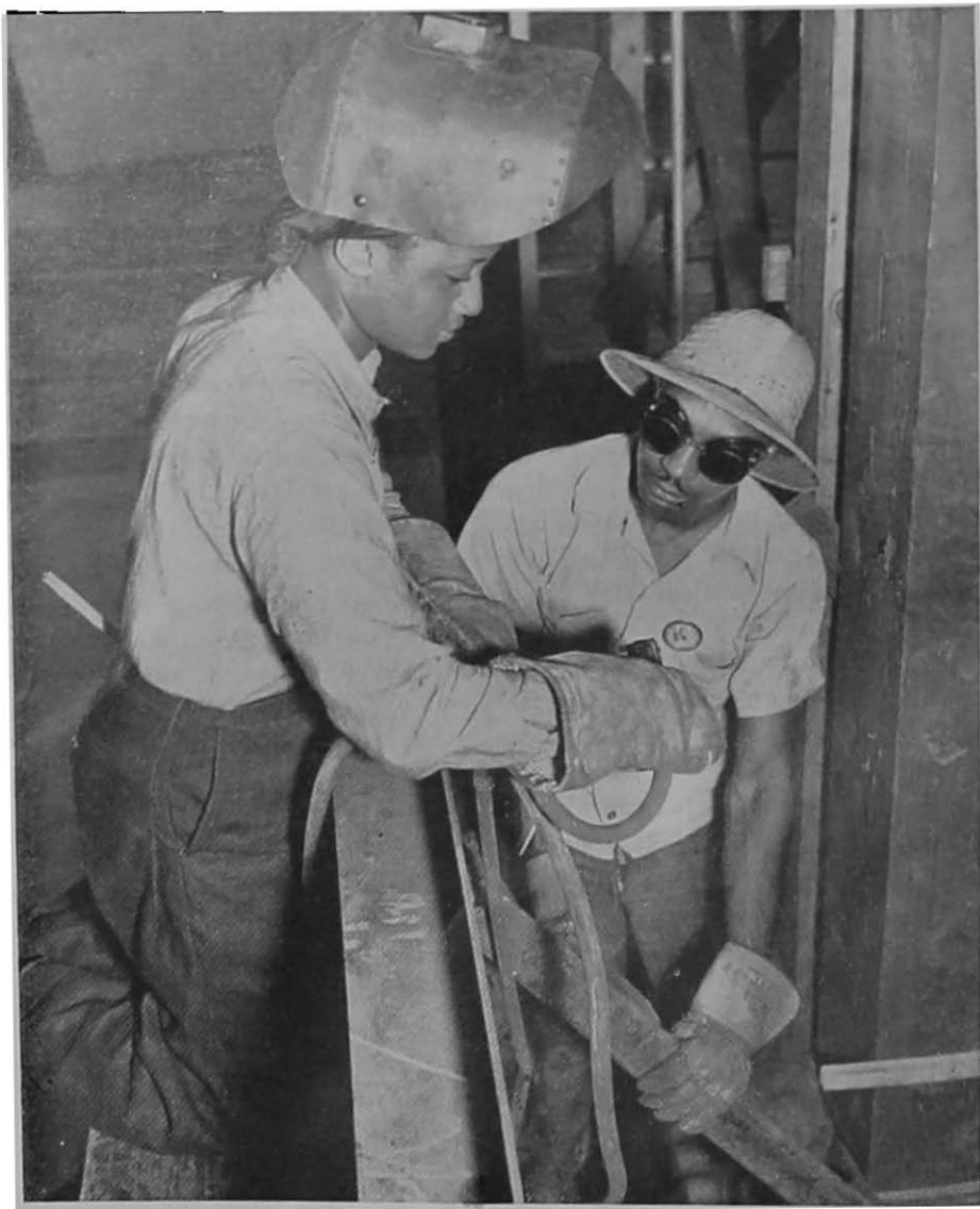
Welder in a shipyard.
