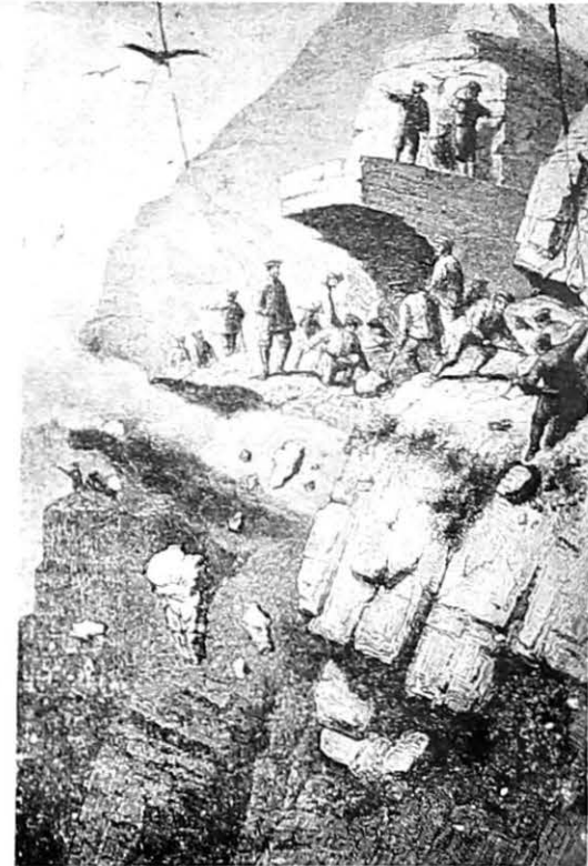
Road Building in the Caucasus, Russia, 1880.
