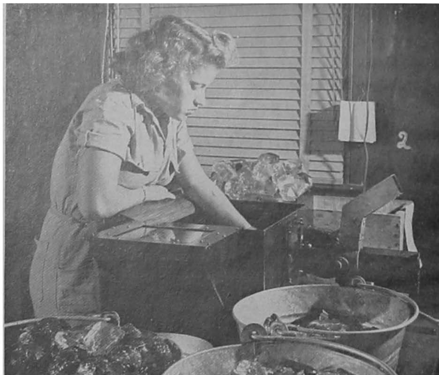
GIRL EXAMINING QUARTZ BY SUBMERSING THE CRYSTAL IN A MINERAL OIL BATH.
