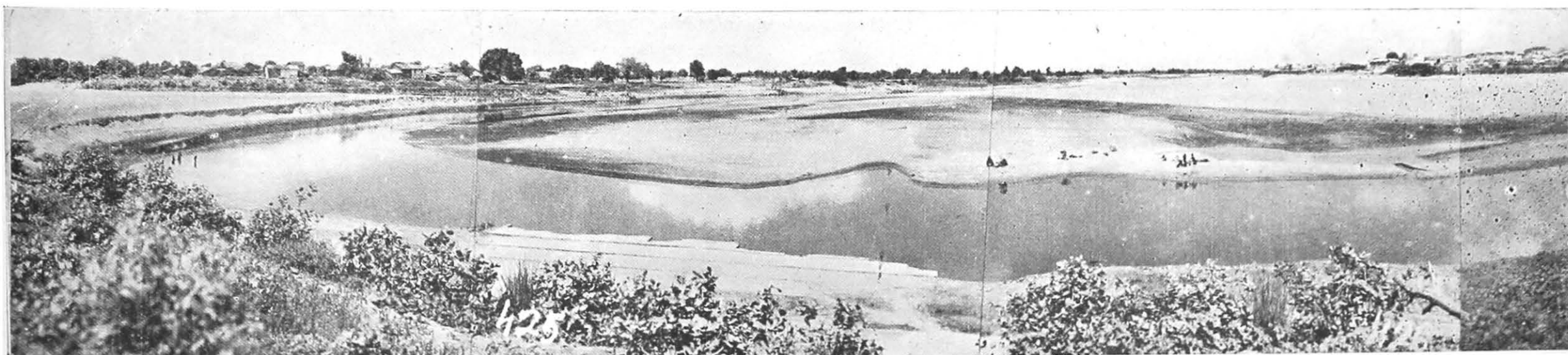
Photo Nos: 424 427 Looking upstream of the Road Bridge showing Hariala Village, tree groynes and the river channel along right bank; fort wall and Kaira Town on left bank. Note parallel flow of the river along approach embankment seen in foreground.
