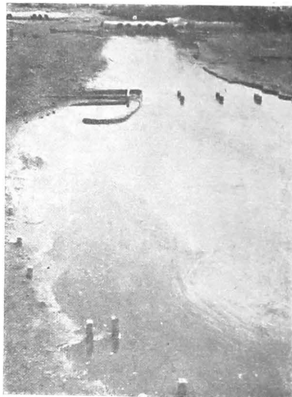
Photo No. 64-Looking down-stream showing high flood discharge with the guide bund aligned as per drawing No. 11425 24. F.
