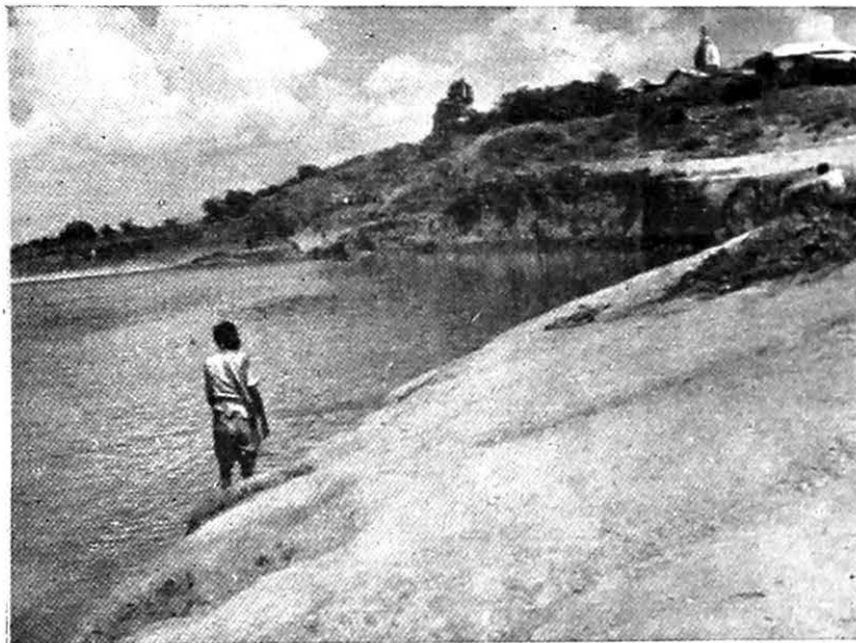
Photo No. 422 The left bank, along the bend, under erosion with Hanuman Temple on a hillock in the background.
