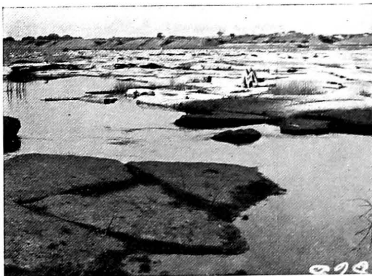
Photo No. 828 River bed in the vicinity of the proposed Barrage is strewn with big rocks.
