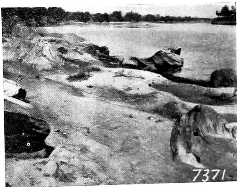
Photo No. 7371 Subernarekha river Jamshedpur. River bank upstream of pump house.
