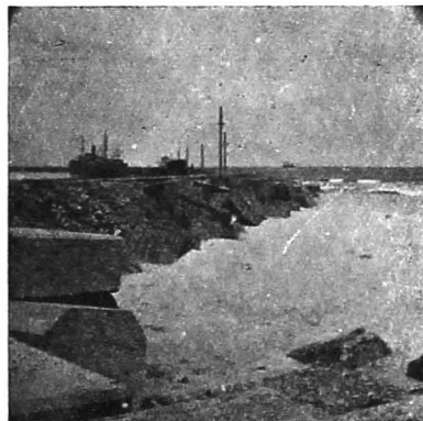
Photo No. 5329—Showing accretion between east Quay and projecting arm of South Quay. Concrete blocks as wave breakers in the foreground.
