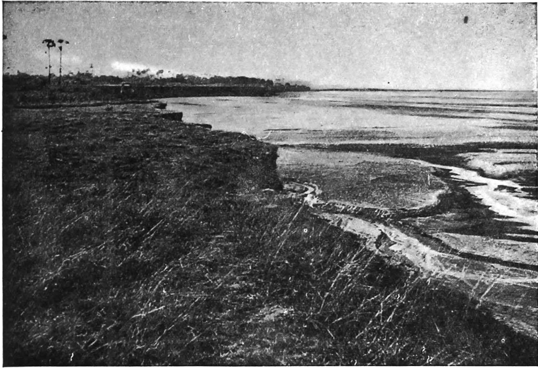
Photo No. 5578—Gautami River 200 feet above right abutment showing steep scoured bank looking upstream.
