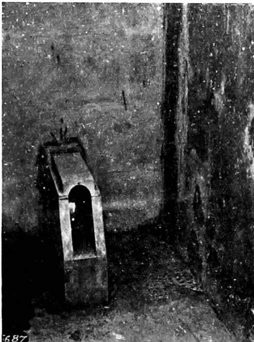
Photo No. 5687—Showing downstream view of the sluice model—Radhanagari Dam Works.
