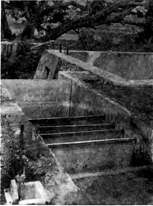
Photo No. 5666—Showing end of the approach channel with grids for equalisation of velocities and ensuring smooth flow.
