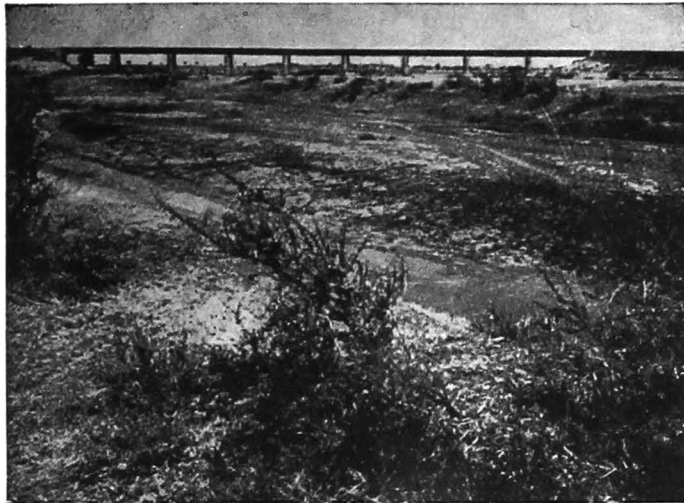
Photo No. 5525-Showing the Radihalla approach to the Railway Bridge.
