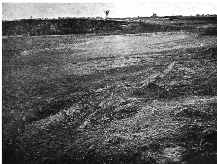
Photo No. 5530- Showing the developed cut from Bennihalla to Radihalla.
