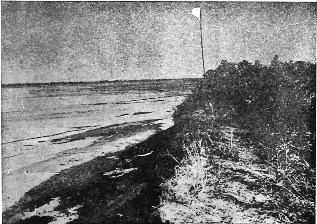
Photo No.5580—Proposed site of Gautami Bridge (right abutment) flaggcd pole on centre line on Bridge.
