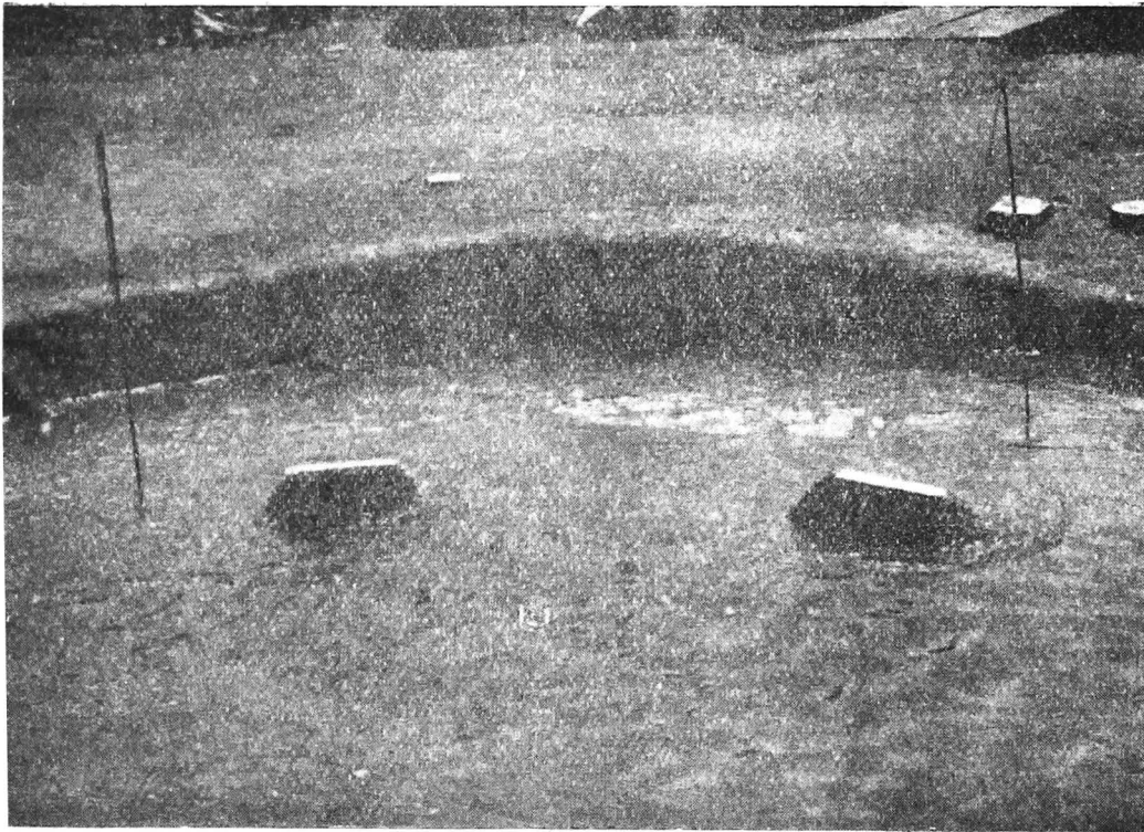
PHOTO No. 5226. Two pitched islands in relation to the infiltration gallery alignment represented by the rods.
