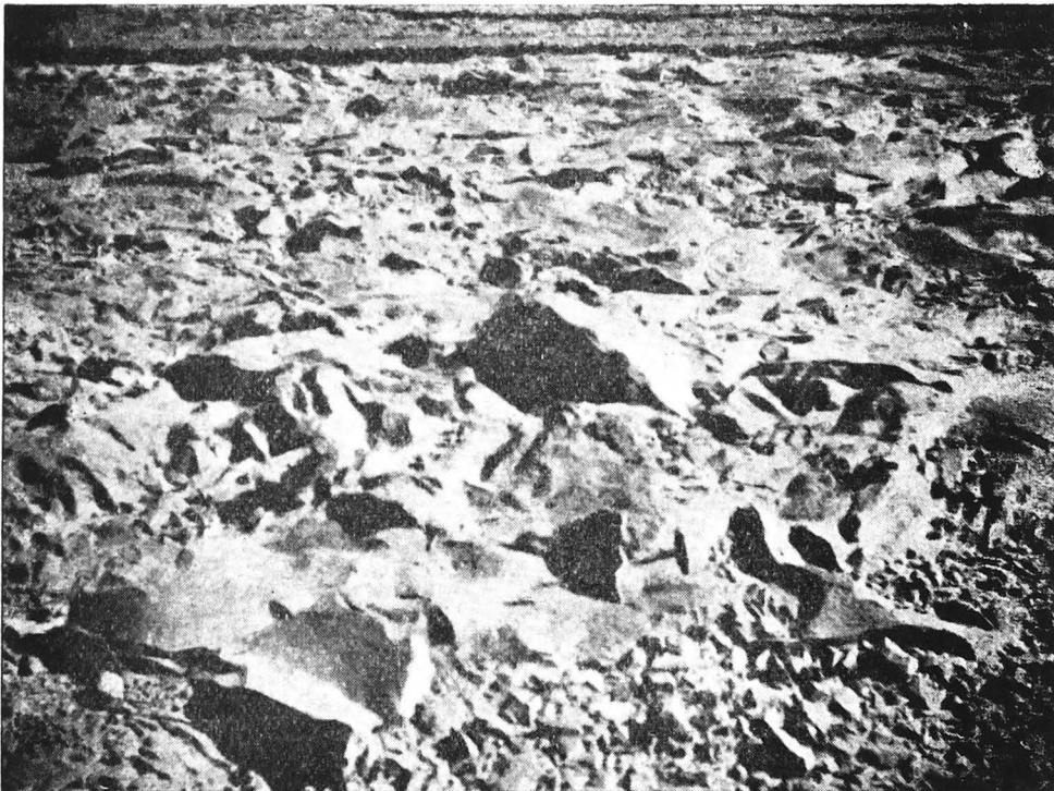
PHOTO No. 1295. Photograph showing downstream portion of weir on Left Bank.
