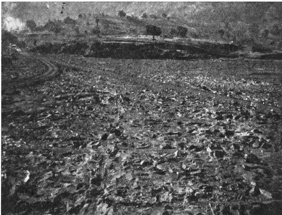
PHOTO No. 1296. Photograph showing downstream portion of weir on Right Bank.
