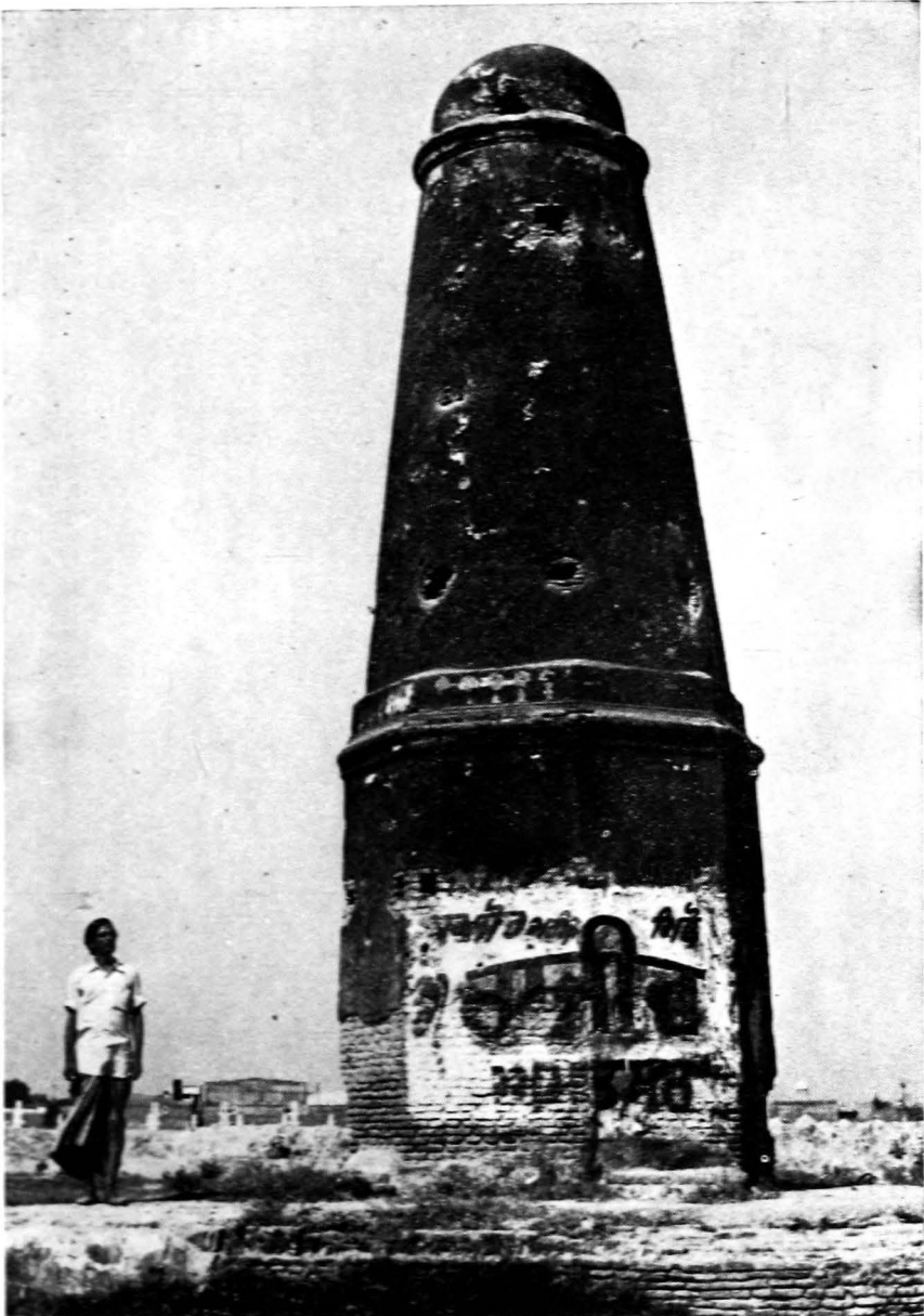
FIG. 51. A kes-minar near Ludhiana, 1960. Such minars were constructed at a distance of a kes (about 3.2 kilometres, or 2 miles) along the Grand Trunk Road from Lahore to Delhi by Jahangir. In the niches oil lamps were lighted at night to guide the travellers.
