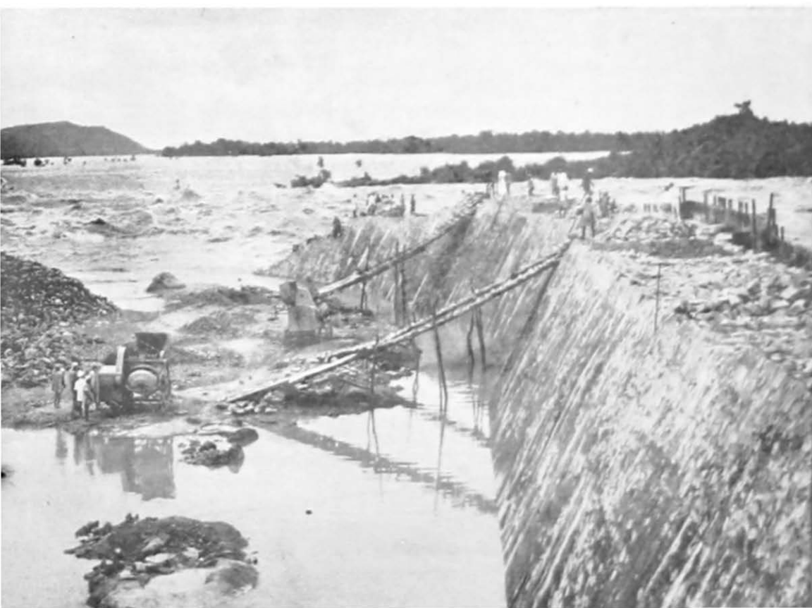
Hirakud Project. Left flank wall under construction
