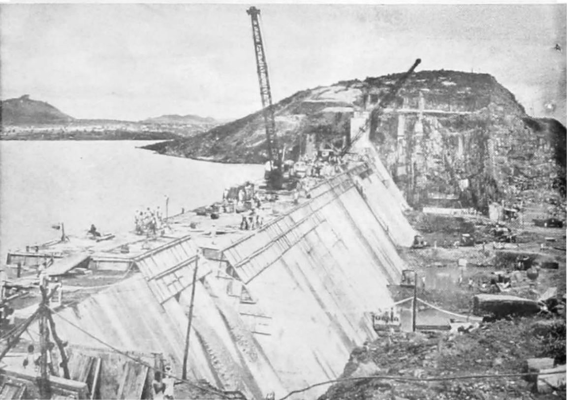
Damodar Valley Project. Tilaiya dam under construction
