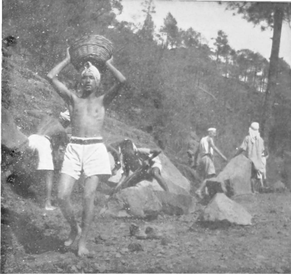
Road building by voluntary workers
