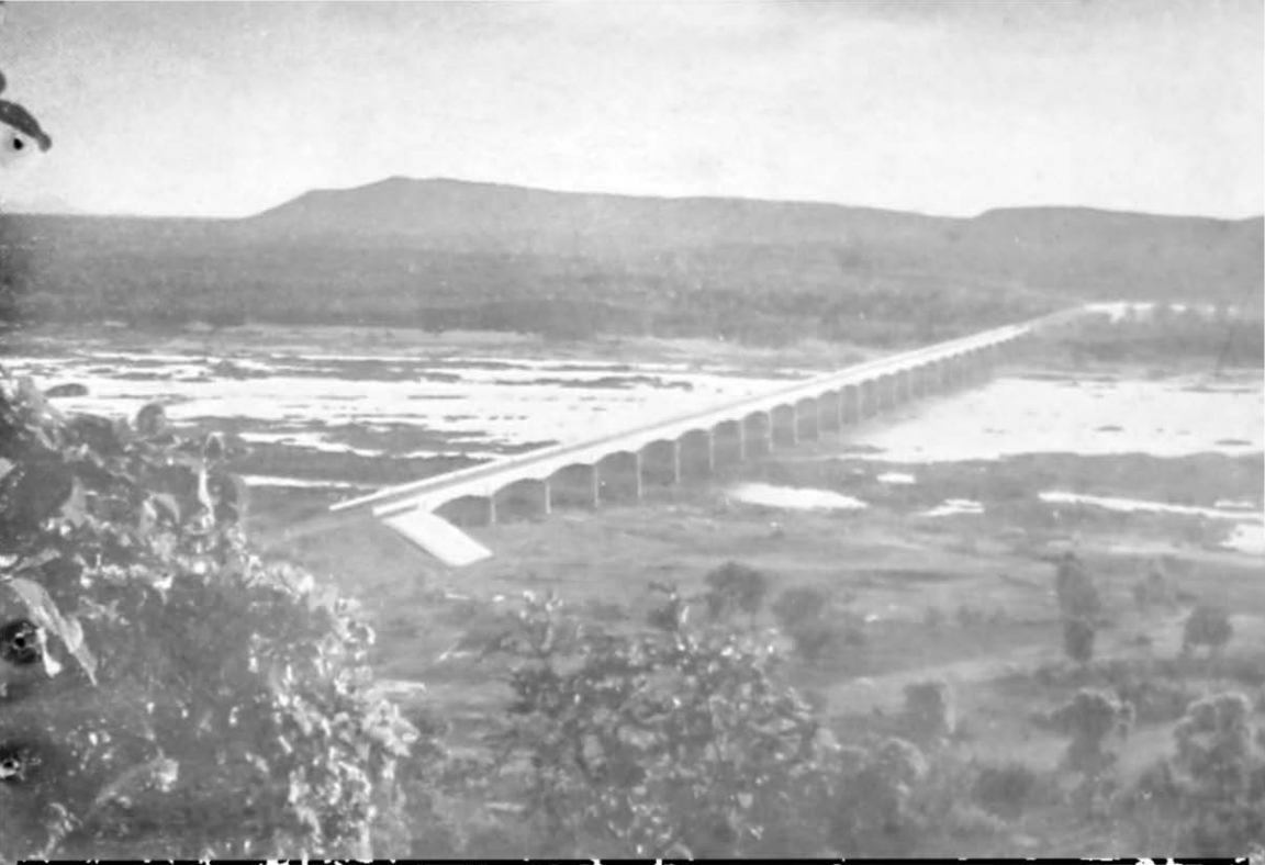
Hirakud Project. Railway and road bridge over the Mahanadi river
