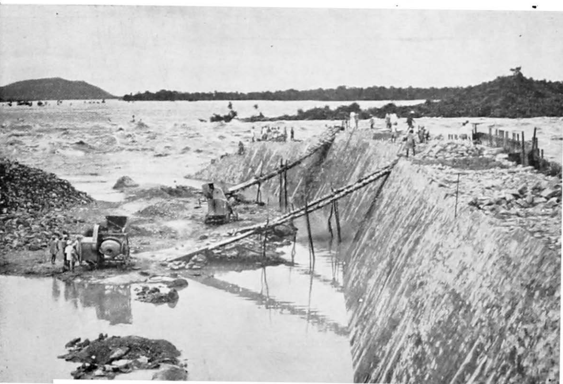
Hirakud Project. Left flank wall under construction
