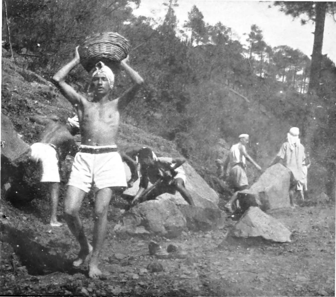
Road building by voluntary workers
