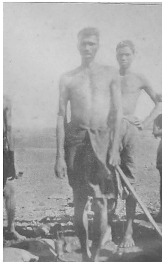
COAL GETTERS STARTING NEW CUTTING.
