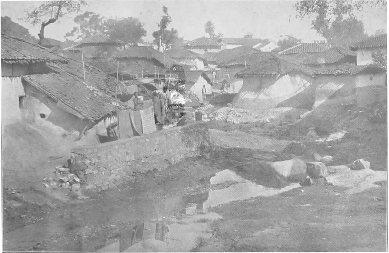
A TEXTILE WORKERS' VILLAGE, SHOWING OPEN DRAIN.
