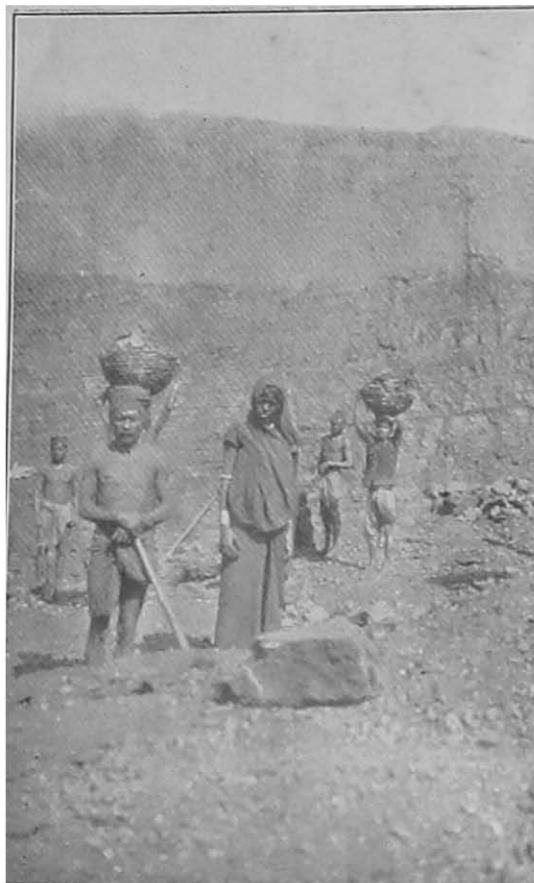
OPEN WORKING: THE THICKNESS OF THE SEAM CAN BE PARTLY OBSERVED.
