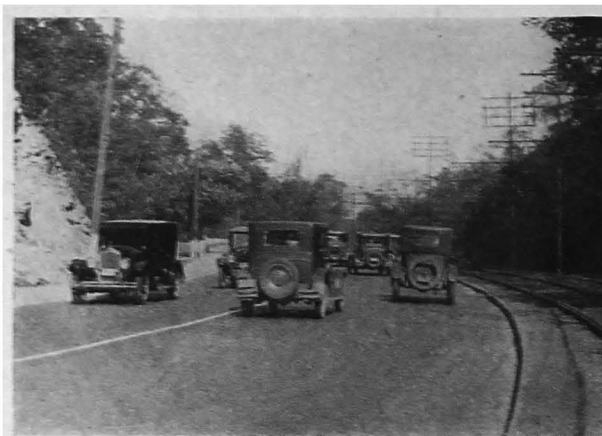
Traffic on congested Cedar Glen Road
