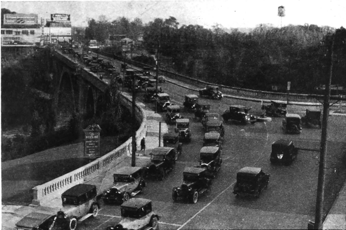
Traffic on the Rocky River Bridge at 3 p. m., Sunday, October 23, 1927. Between 5 and 6 p. m. traffic on this bridge reaches an hourly maximum of more than 2,500 vehicles
