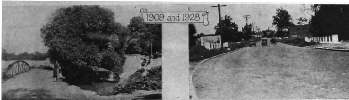
The Euclid Creek Bridge on Lake Shore Boulevard
