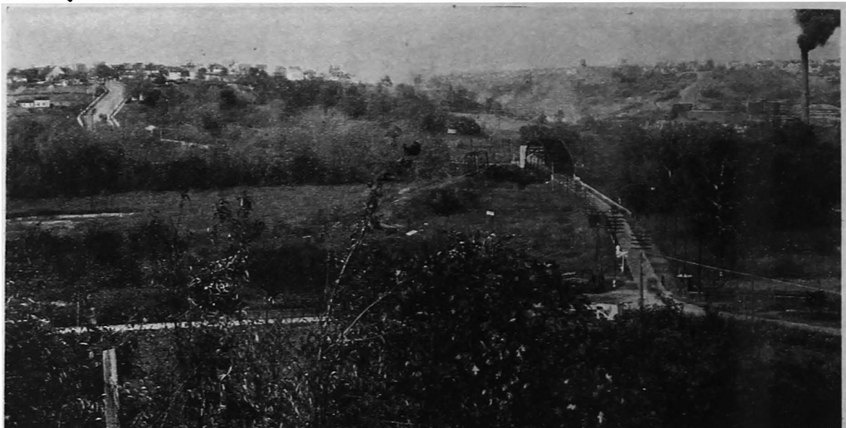
View of Cuyahoga River Valley, at Willow, looking north, showing present location of Brecksville Road and bridge. The relocation of Brecksville Road will pass through the point from which the picture is taken on a direct line to the foot of East 71st Street (upper left). At this point a circular intersection is to be established, serving Brecksville Road and East 71st Street, Brook Park Road (a new East-West Route north of the Cuyahoga River) and the relocation of Independence Road
