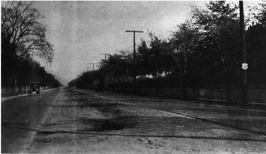
MAYFIELD ROAD NEAR LEE ROAD
