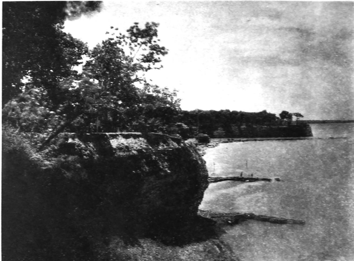
SITE OF THE LAKE-FRONT CROSSING OF ROCKY RIVER
