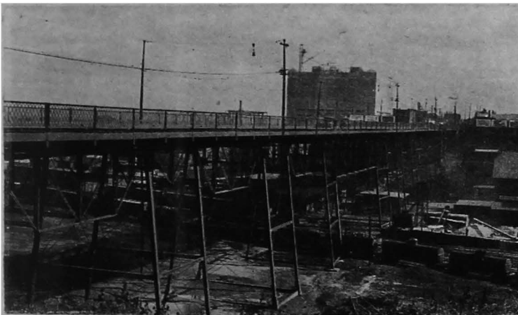
ABBEY AVENUE VIADUCT OVER THE BIG FOUR AND NICKEL PLATE RAILROADS AND SCRANTON ROAD
