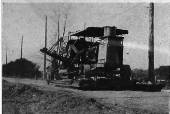
A trenching machine being moved over the highway—an unusual type of load
