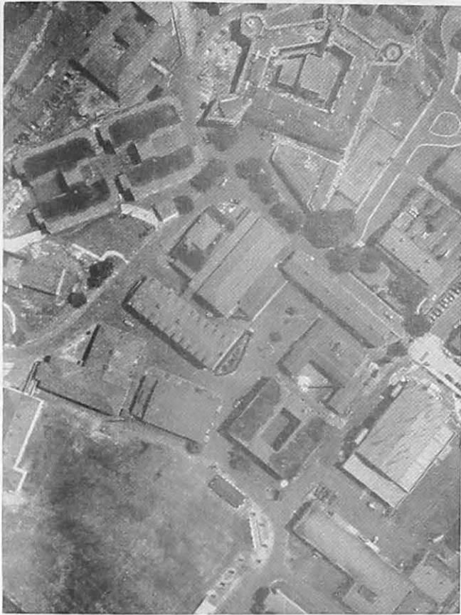
Aerial view, United States Maritime Service Officers' School Fort Trumbull, New London, Conn.
