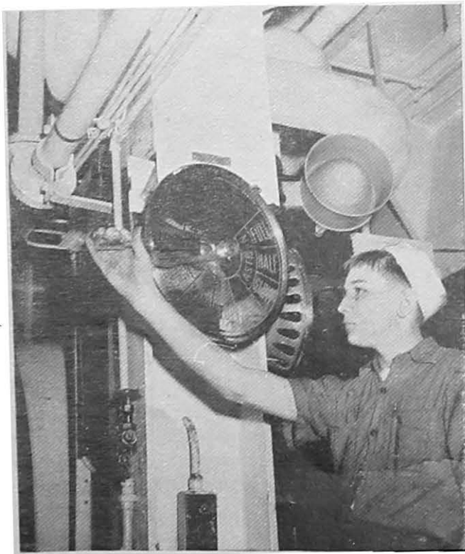
USMS trainee in the engine department receiving practical experience in handling the engine control telegraph. Average training cruise is about 2 weeks
