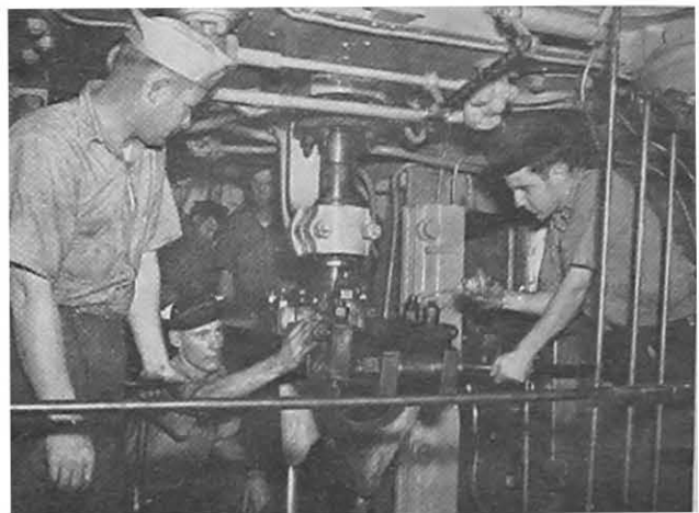
Engineer class of trainees receiving practical experience in oiling and wiping moving parts of machinery
