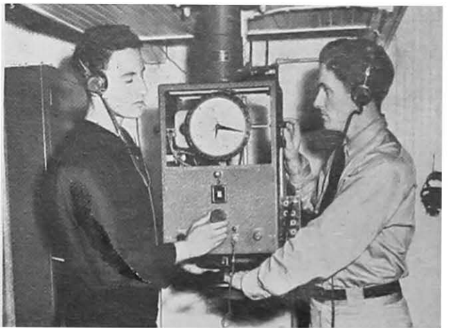
Instructor teaching enrollee method of using ship's radio direction finder for taking bearings
