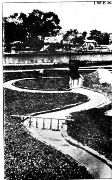
Photo H. 1454. Demonstration model of the Malaprabha River—to show effect of downstream cut-off on flow which threatened to undermine left bank abutment. Three alternative solutions demonstrated—see A. R. (T) 1942-43 pp. 10, 11
