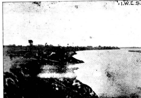
Photo 2607. Sheared bank resulting from deep scour at Dalarghat on Katjuri just downstream of Surua junction with Katjuri. Looking downstream.
