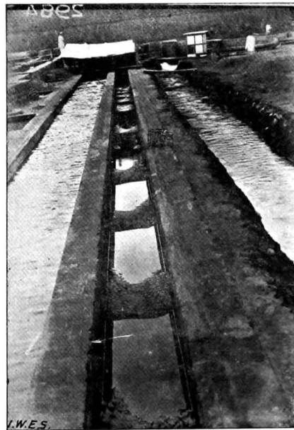
Photo 2984. Dunes in 2\frac{1}{4} ft. channel carrying 5 cusecs.
