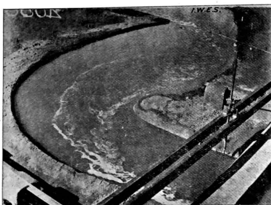
Photo No. 4000. Rupnarain River tidal model. Horizontal scale 1/650. Vertical scale 1/90.
