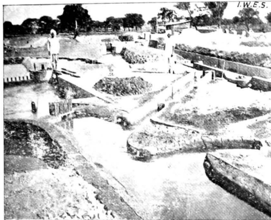
Photo 838. Experiment No. 2 (looking downstream). A spur projecting to midstream was built at the downstream end of the Mithrao to create curved flow to exclude bed sand.
