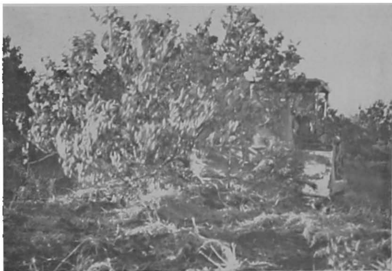
Figure 8. Fruit Tree Being Pushed Out by Bulldozer.
