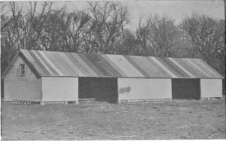
Fig. 1. Roofing samples in place for weathering tests.
