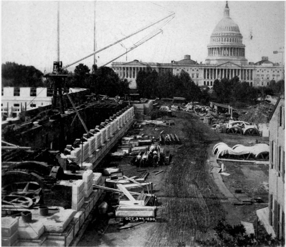
Construction of the Main Building of the Library of Congress, which required eight years, from 1889 to 1897, is pictured here at an early stage. Of monumental structure and artistic perfection even to minute details, the building was erected under the direction of Brigadier General Thomas Lincoln Casey, Chief of Engineers, United States Army.
