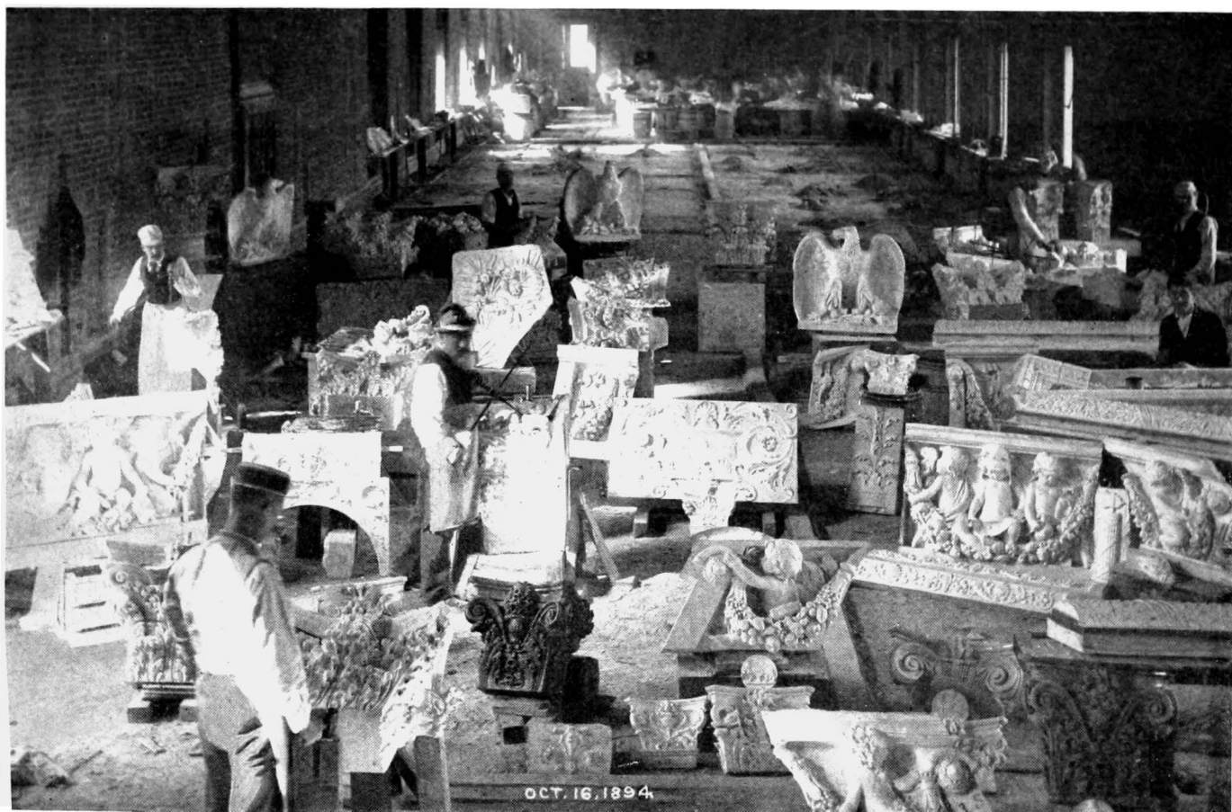
Decorative work for the new Library building. Taken October 16, 1894, this photograph shows marble cutters and other artisans preparing material which later was embodied in the friezes and other ornamentation of the Main Building.
