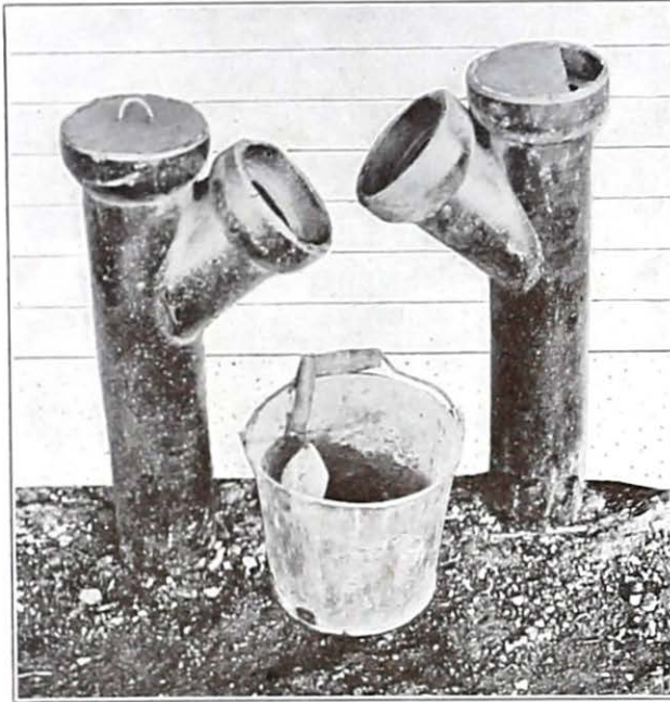
Fig. 7. —Plugs placed in inlet and outlet Y's according to Step 3. Tin or tar paper circles in the bottom of the bell hold the mortar in place. A dam makes the vent with the edge of the disk turned up in outlet piece at right.
