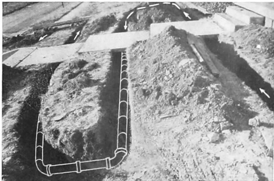
Fig. 13. —Four straight runs of absorption tile in a front yard connected by cemented sewer pipe joints and elbows at turns down hill. See front cover.
