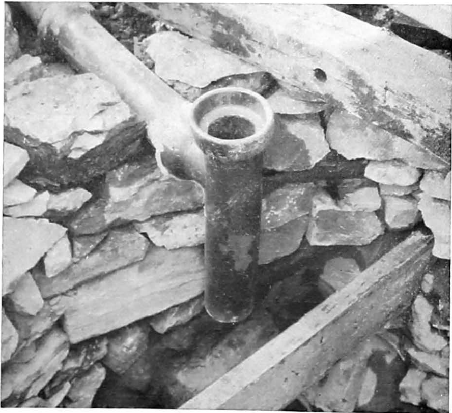
Fig. 17. —A sewer pipe "T" cemented to a straight piece of 4-inch sewer pipe and hung vertically to serve as an outlet for a cesspool. Figure 19 also shows this between the two chambers. The wall was built up higher. More baffle was added to keep the scum from entering the bell when it gets thick. This procedure is only adapted to locations where the water supply cannot be contaminated.
