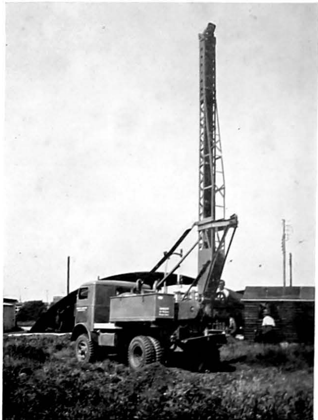
(B) POWER AUGER SUITABLE FOR BORING IN GRAVELLY SOILS
