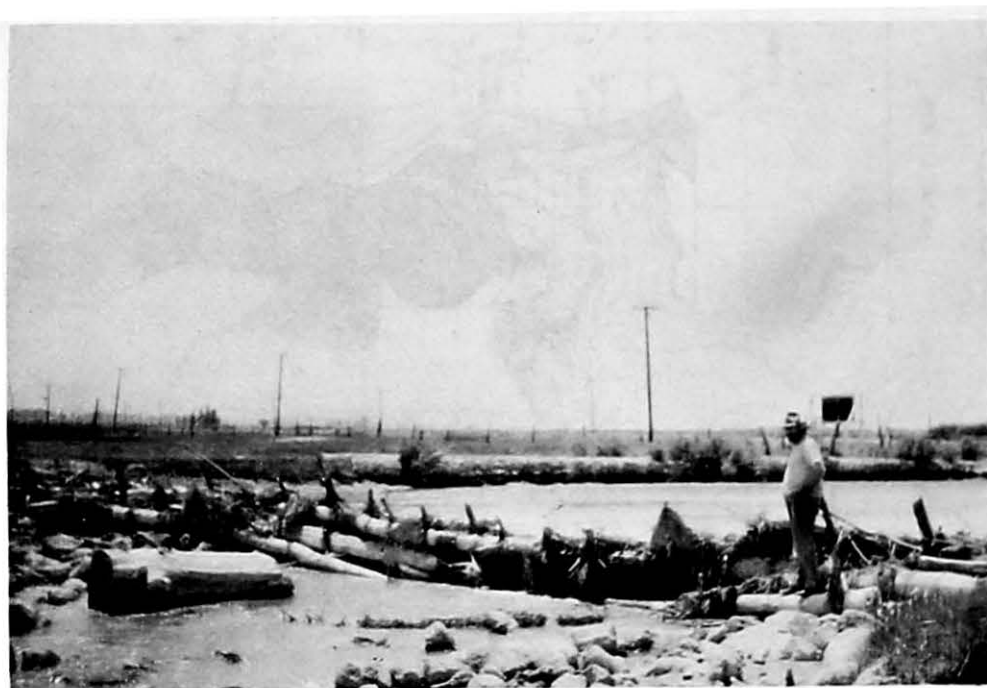
Fig. 5. West view Canal Company's Diversion Dam, diverting water from the Sevier River. Typifies needed replacement of inadequate diversion structures.
