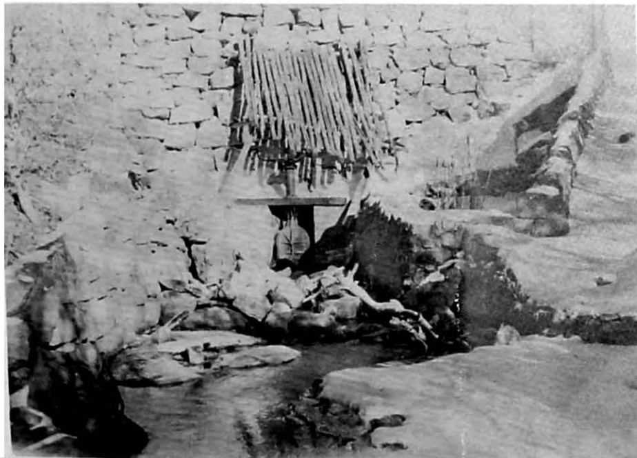
Fig. 4. Lower Bell Canyon Reservoir Dam, Salt Lake County. Typifies dam and outlet works requiring repair or replacement.
