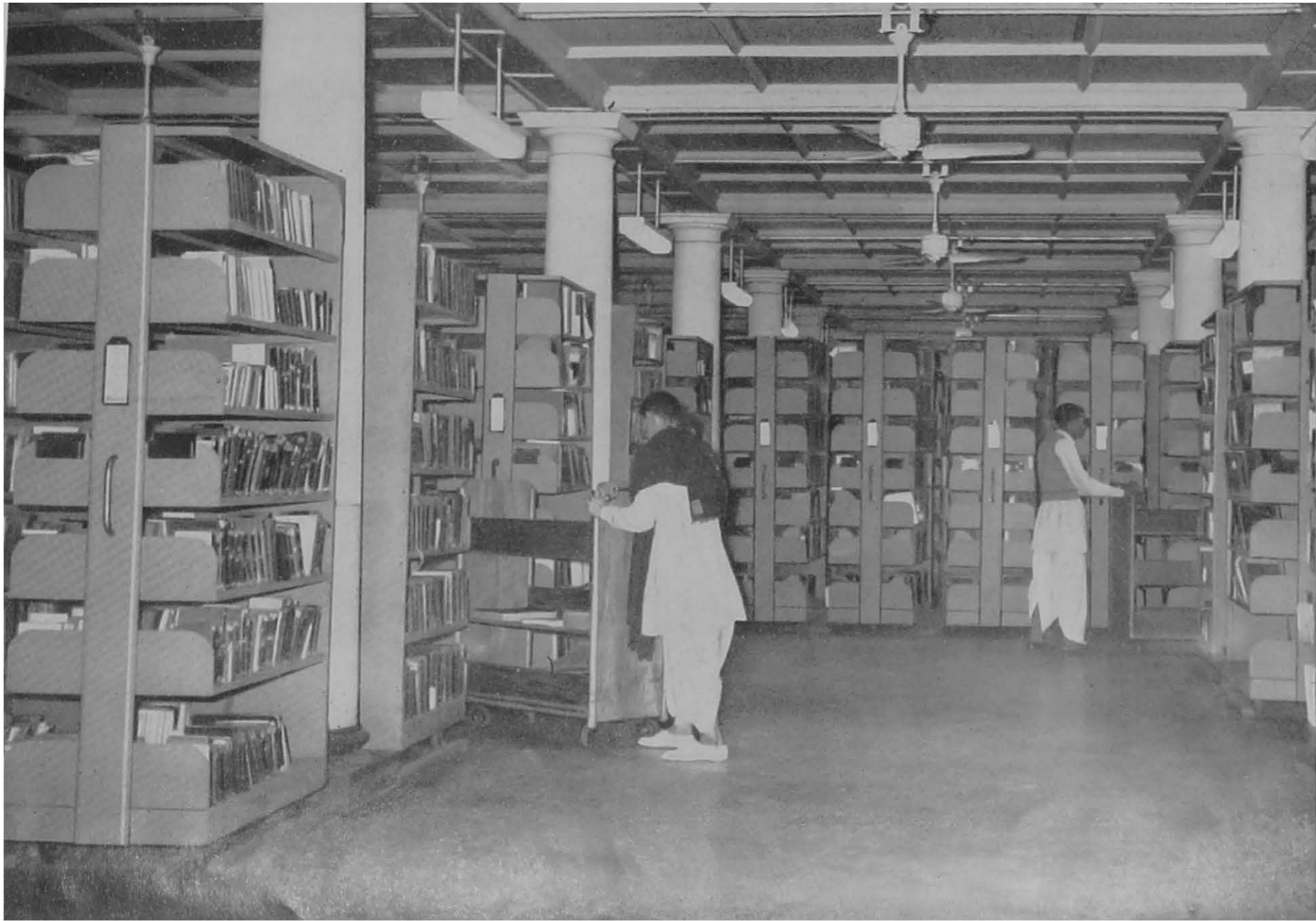
PLATE 8. The stack room as seen from the east entrance. The rolling stacks, the first of their kind in India, have been designed to save space, to isolate books from termites, etc., to facilitate easy cleaning, and to allow their being shifted about easily. The easy guiding of these stacks is quite a feature of the design.
