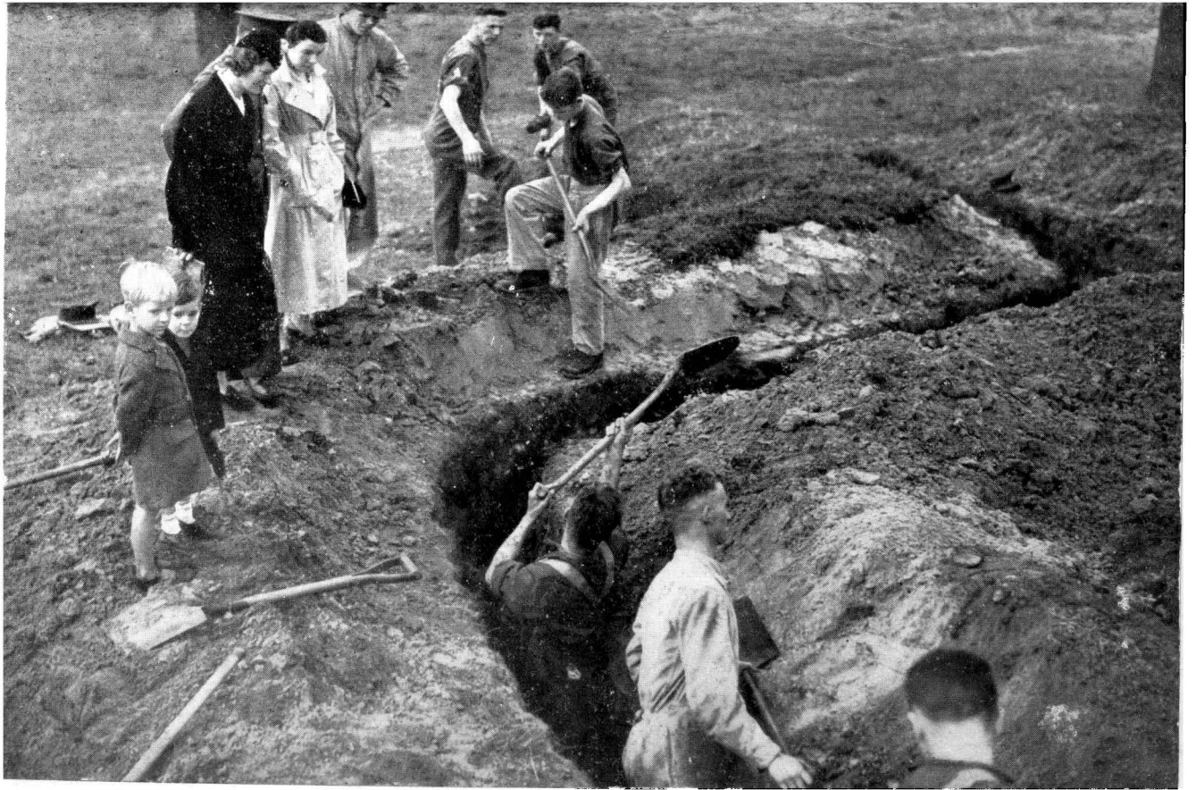
Trenches being hastily dug at Aldershot, England in Sept., 1938. Note the zig-zag formation.
