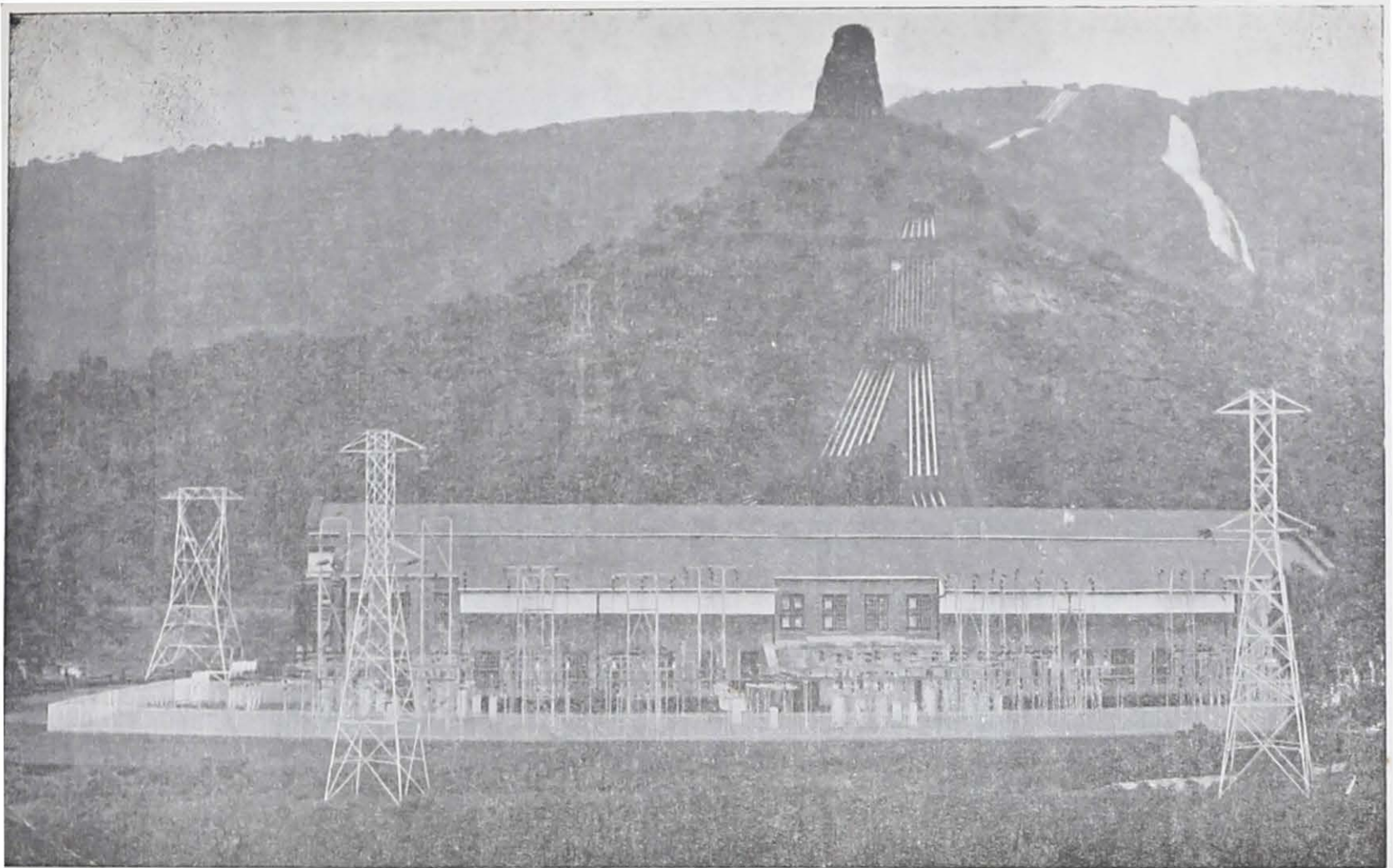
Bhira Power House and Pipe Line
