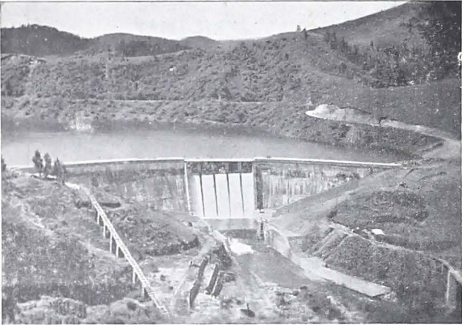
Pallivasal Hydro-electric Project—Sethu Parvathi Poran Dam
