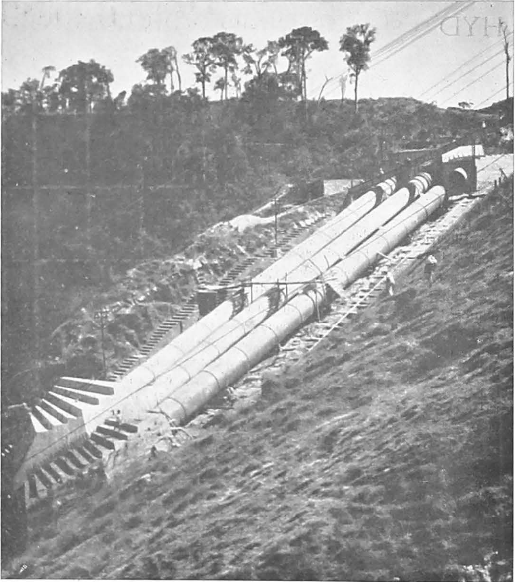
Mahatma Gandhi Hydro-electric works—Pipe line middle section.
