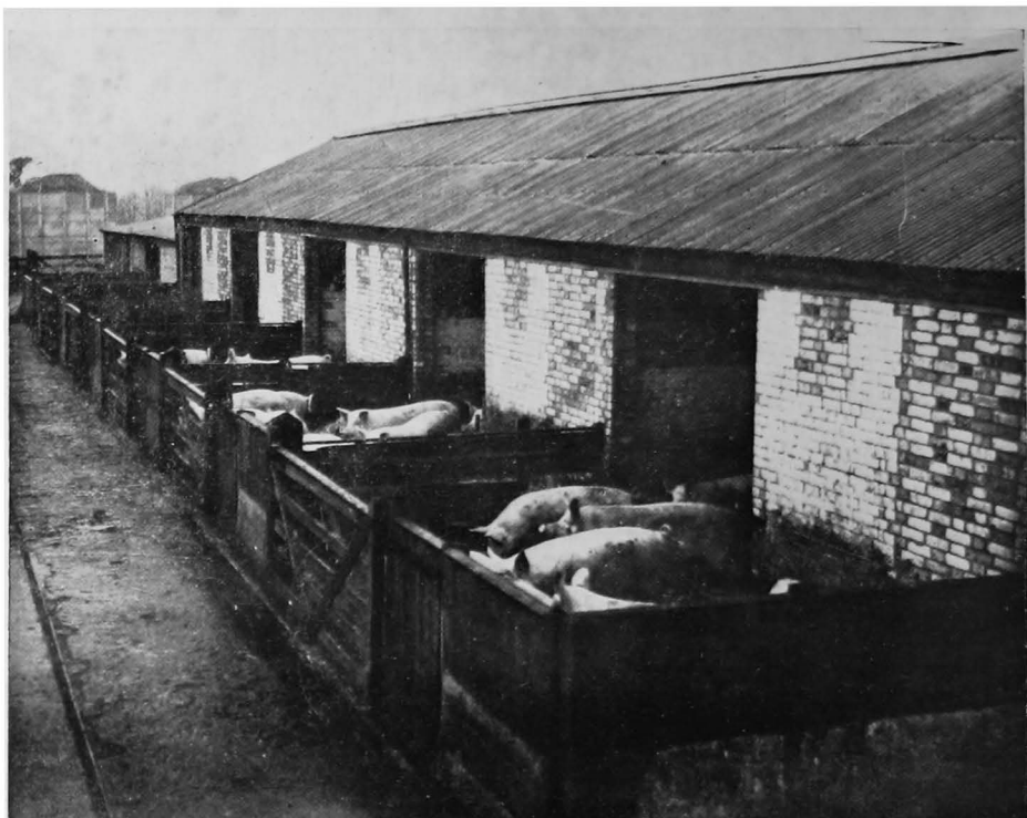
PLATE 13. RANGE OF STIES WITH YARDS ADAPTED FROM DRAUGHTY DOUBLE-RANGE PIGGERY Formerly pigs did badly, now they do well. Note shutters for controlling ventilation lowered in bottom two yards.
