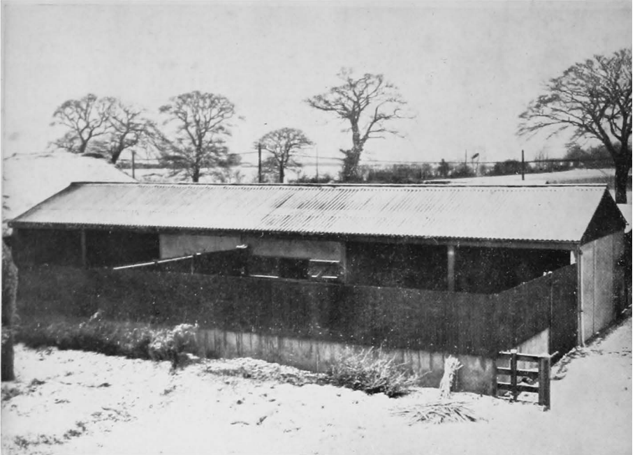
PLATE 7. HORSE YARDS FACING SOUTH AND SHELTERED BY HIGH FENCE Can be easily adapted for cattle. The centre section is a harness room, chaff house, and food store.
