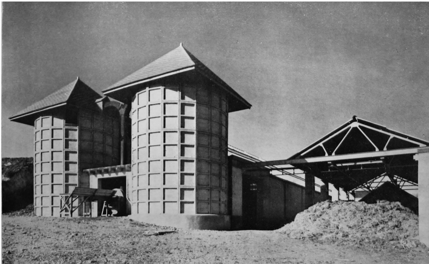
PLATE 2. A MODERN FARMSTEAD IN SOMERSET: SILOS, COWHOUSE, AND DUNGSTEAD Note fixed blower and conveyor.
