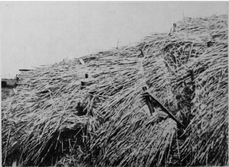
PLATE 22. STRAW ROOF HELD DOWN BY BALING WIRE AND THATCHING PINS
