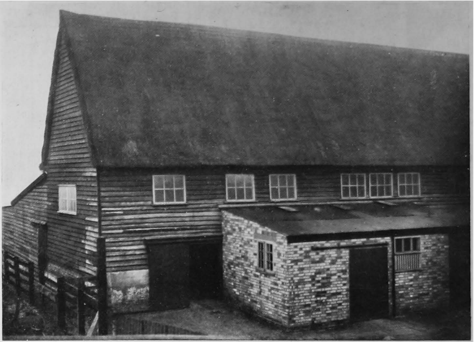
PLATE 5. ADAPTATION OF BARN INTO MILKING SHED AND OPEN YARDS NORTH SIDE: MILKING SHED The new brick building is for milk storage.
