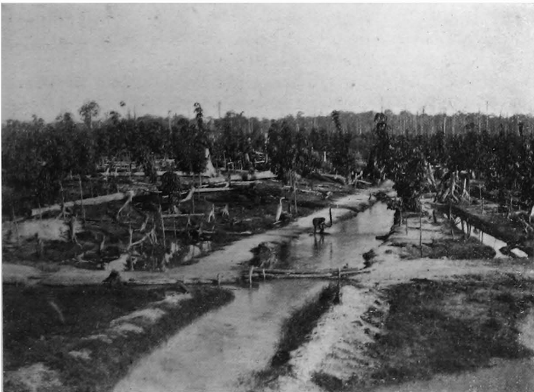
FIG. 75. A Stream too large for Pipe Drainage.
