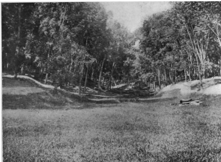
FIG. 34.—SEAFIELD ESTATE, The Ravine of Fig. 32 when finished.
