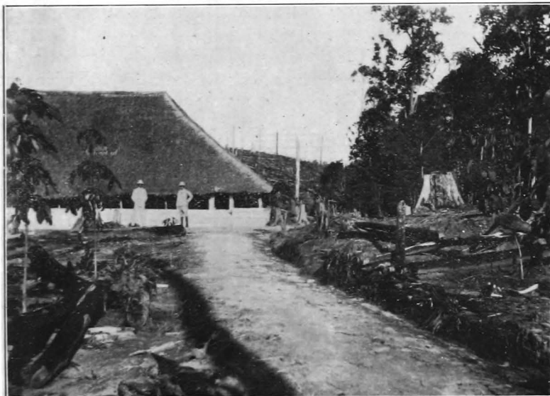
FIG. 85.—MOSQUITO-PROOF COOLIE LINES.
