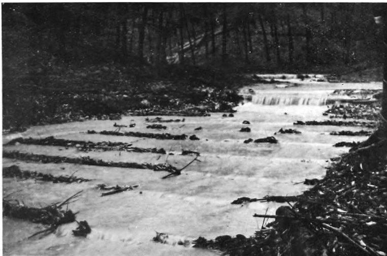
FIG. 39.—SEAFIELD ESTATE. Ravine "A" during a tropical shower, after subsoil drainage.
