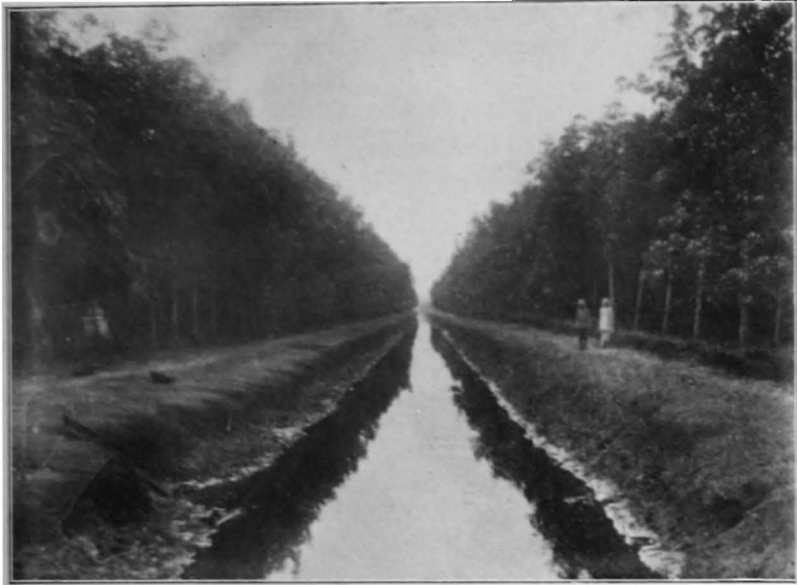
FIG. 12.—KAPAR DRAINAGE SCHEME. One of the main drains, with rubber trees on both sides.
