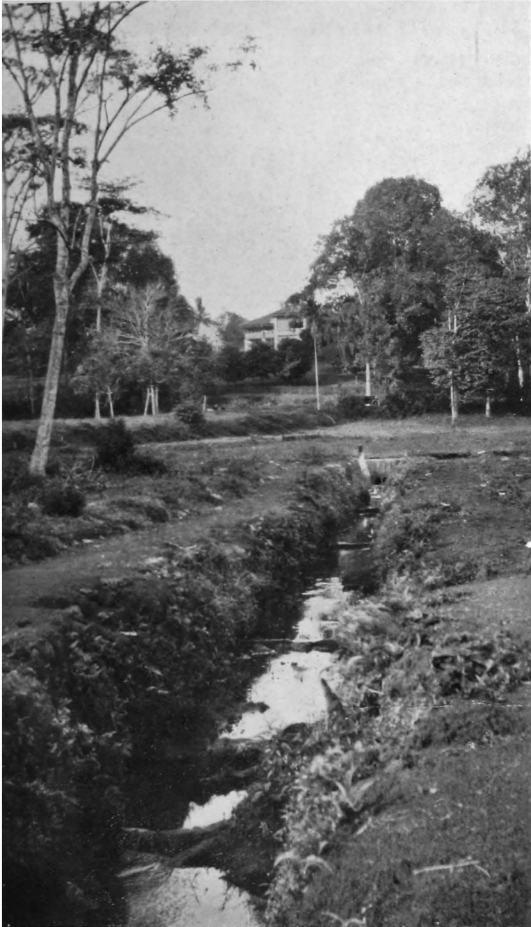
FIG. 108.—SINGAPORE. Open Ditch into which the subsoil drains discharge.
