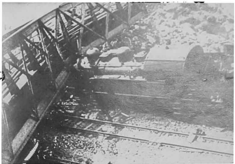
Well trapped! One transport to the East less!
