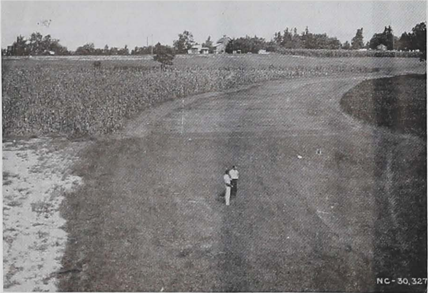
A meadow Strip Outlet prepared and seeded in advance of terracing. Carries the water from 60 acres and produced 7\frac{1}{2} tons of hay.
