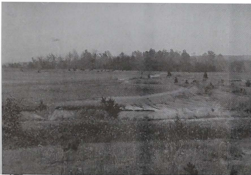
A diversion ditch intercepting water from the area above a badly eroded section, which is to be terraced.
