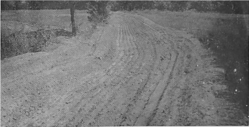
Preparing the outlet for permanent seeding and protection.
