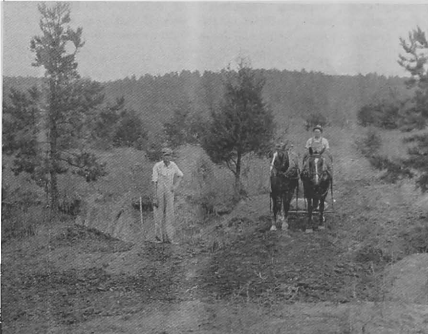
Filling a gully preparatory to constructing a terrace across it.
