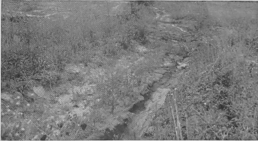
A natural untreated field outlet showing early stages of erosion.
