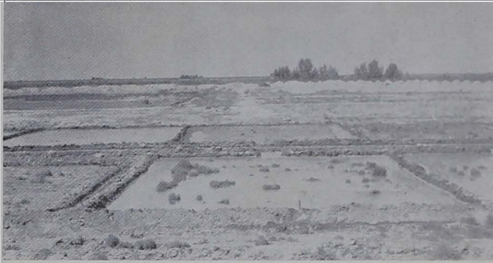
Fig. 5. View of plots at site C during leaching operations
