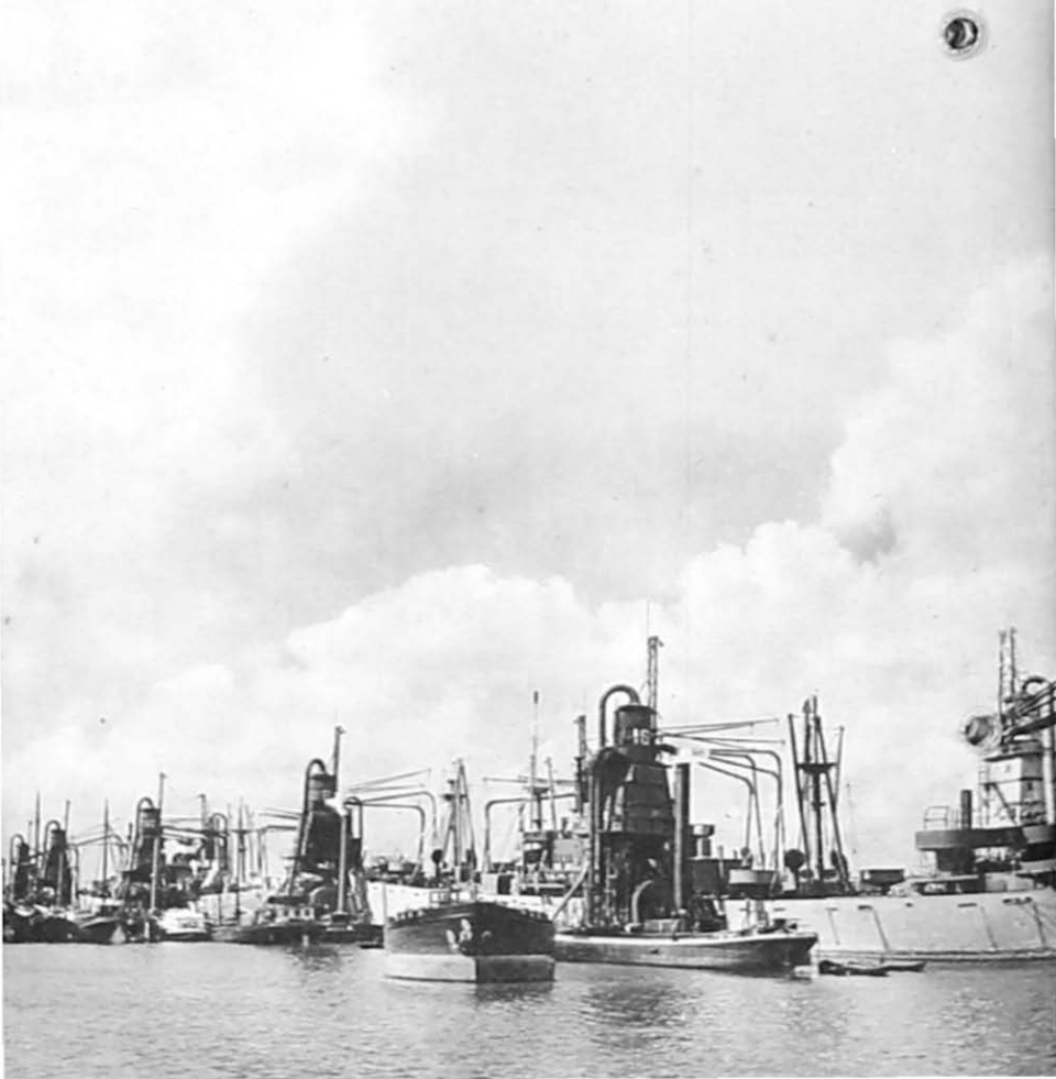
Grain Elevators, Rotterdam
