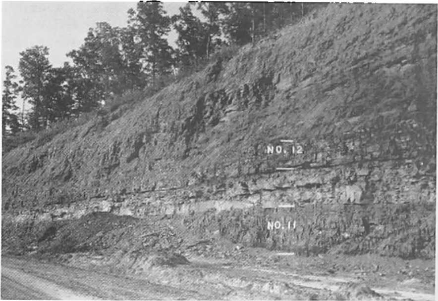
Fig. 10. — Typical high-wall for the No. 11 and No. 12 coal as observed in the Western Coal Field in Hopkins county. The two coal seams are separated by a bed of limestone and clay. The height of wall is about 40 feet. (Homestead Mining Co., near St. Charles, Hopkins county.)
