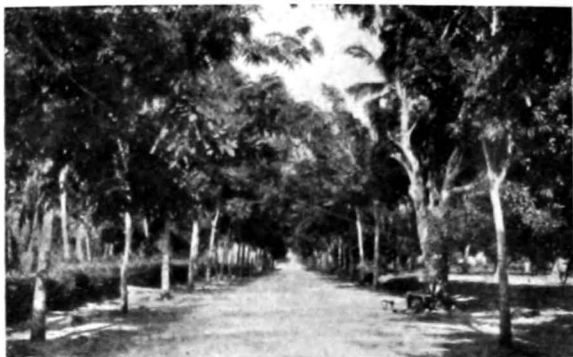
ROAD IN DAR-ES-SALAAM.
