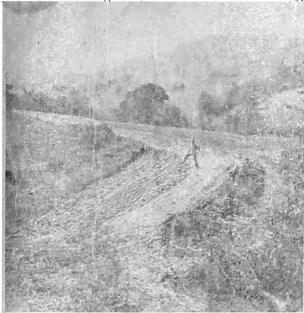
Figure 5.—A diversion just constructed on a long slope on class IV land. Water is to be discharged at right angles to slope into a natural rock drainageway.
