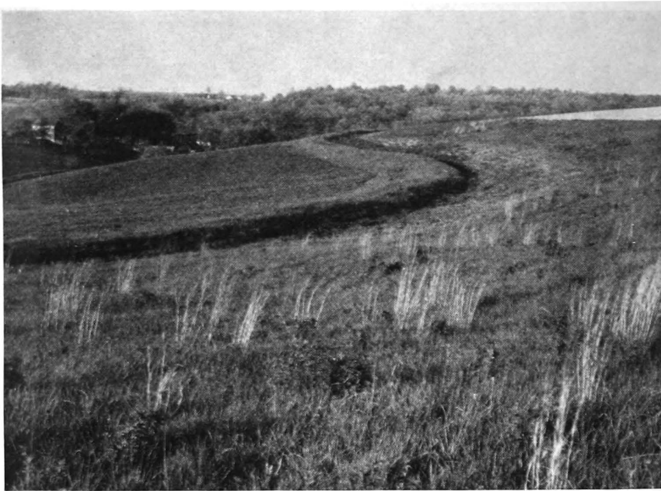
Figure 11. —A diversion terrace breaking a long slope into two shorter ones. Water is carried away on a gentle grade. A grass strip above protects the terrace.
