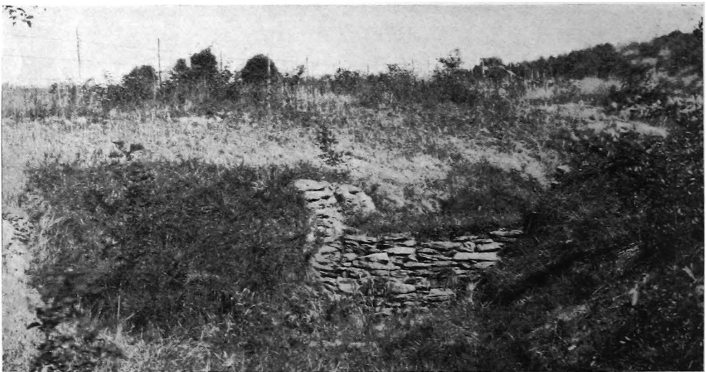
Figure 16. —A temporary check dam in a formerly active gully. The banks are planted to locust; the bottom and sides are seeded to protective grasses. Water flows through the dam, but earth is held in place to fill the gully.
