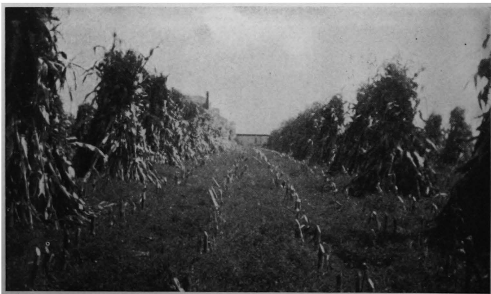
Figure 9.—A cover crop of sweetclover sown in corn affords winter protection against erosion and provides organic manure to be plowed under.
