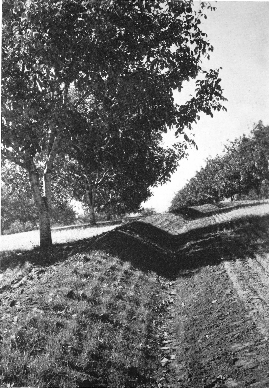
A field diversion-ditch system constructed in a walnut orchard on a 15 to 20 percent slope in Olympic soil. The trees are spaced 60 feet apart.
