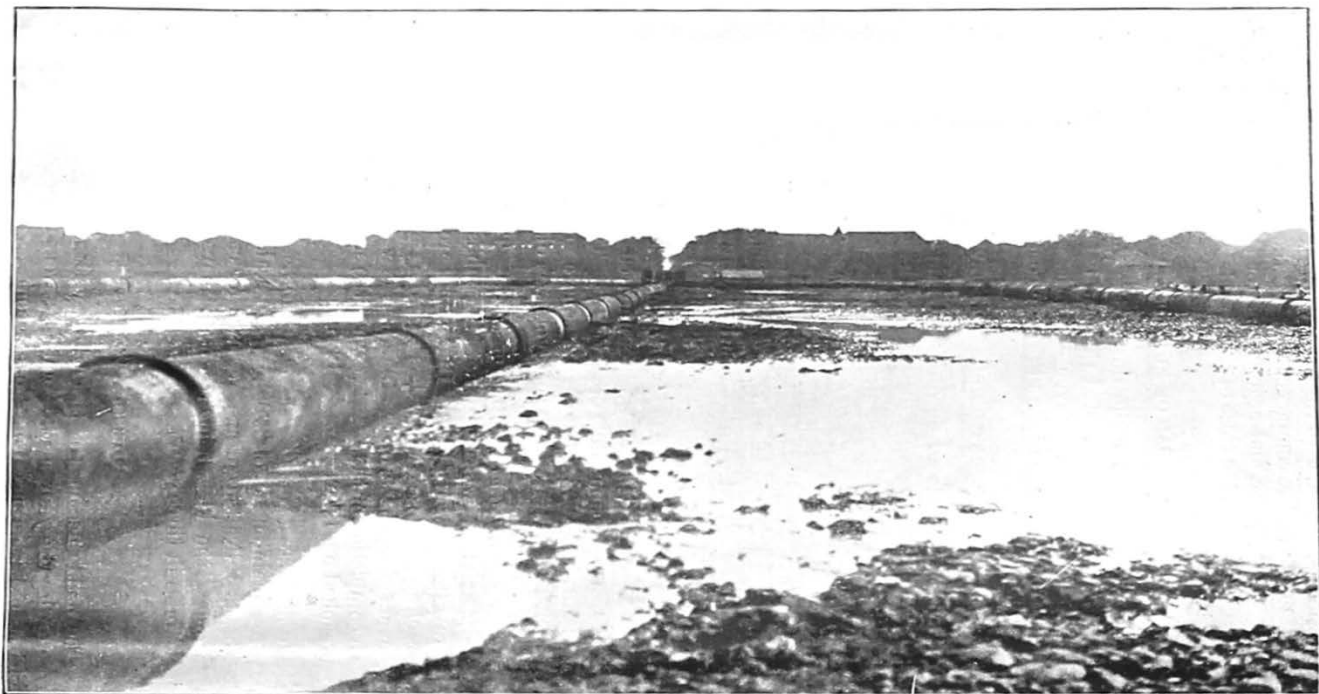
General view showing Area reclaimed. Arrangement of pipes with 3-way piece. 16-12-25
