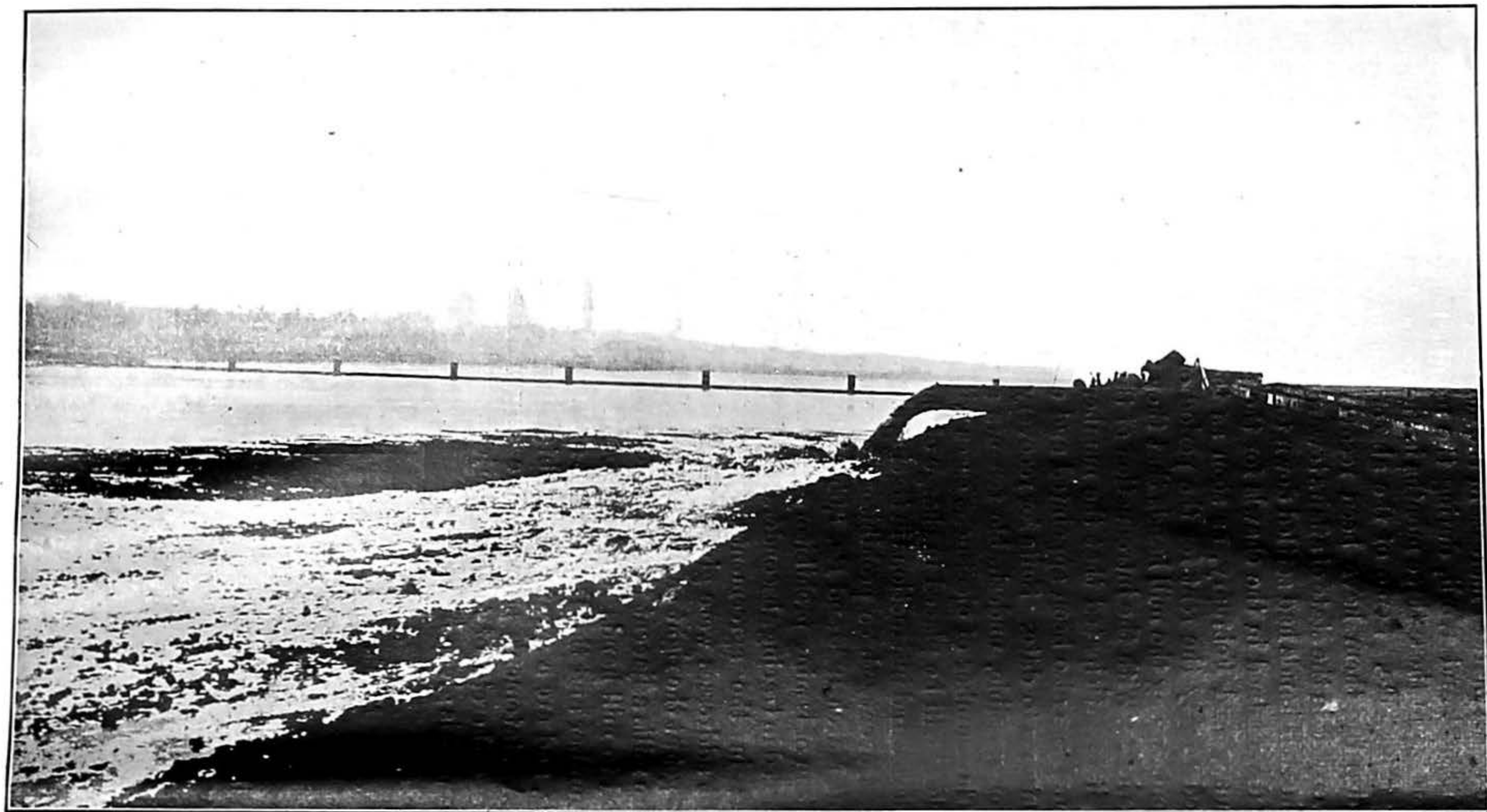
Discharge at Back Bay. 16-12-25
