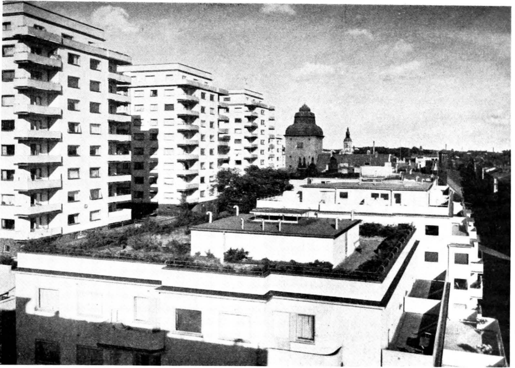
Apartment houses in Stockholm, built and managed by the Stockholm Tenants Building Cooperative Society (H. S. B.).
