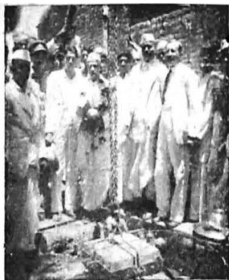
Hon'ble Mr. N. V. Gadgil lays the Foundation Stone on 25-4-49.
