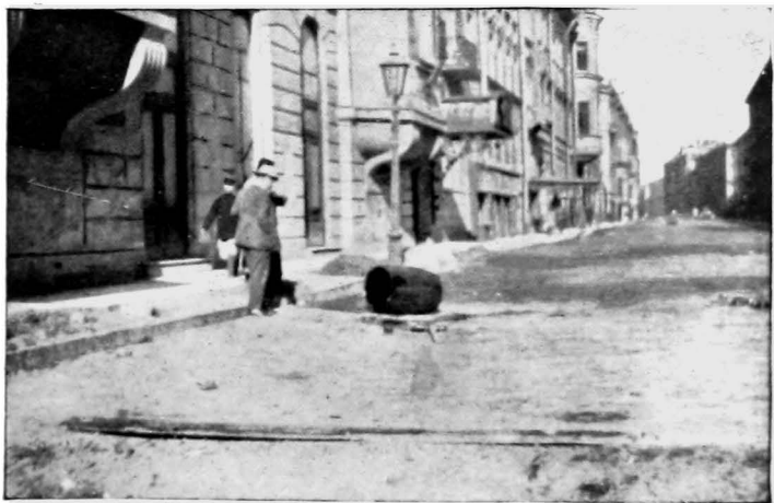
MR. WELLS DISCOVERS A STREET UNDER REPAIR.
