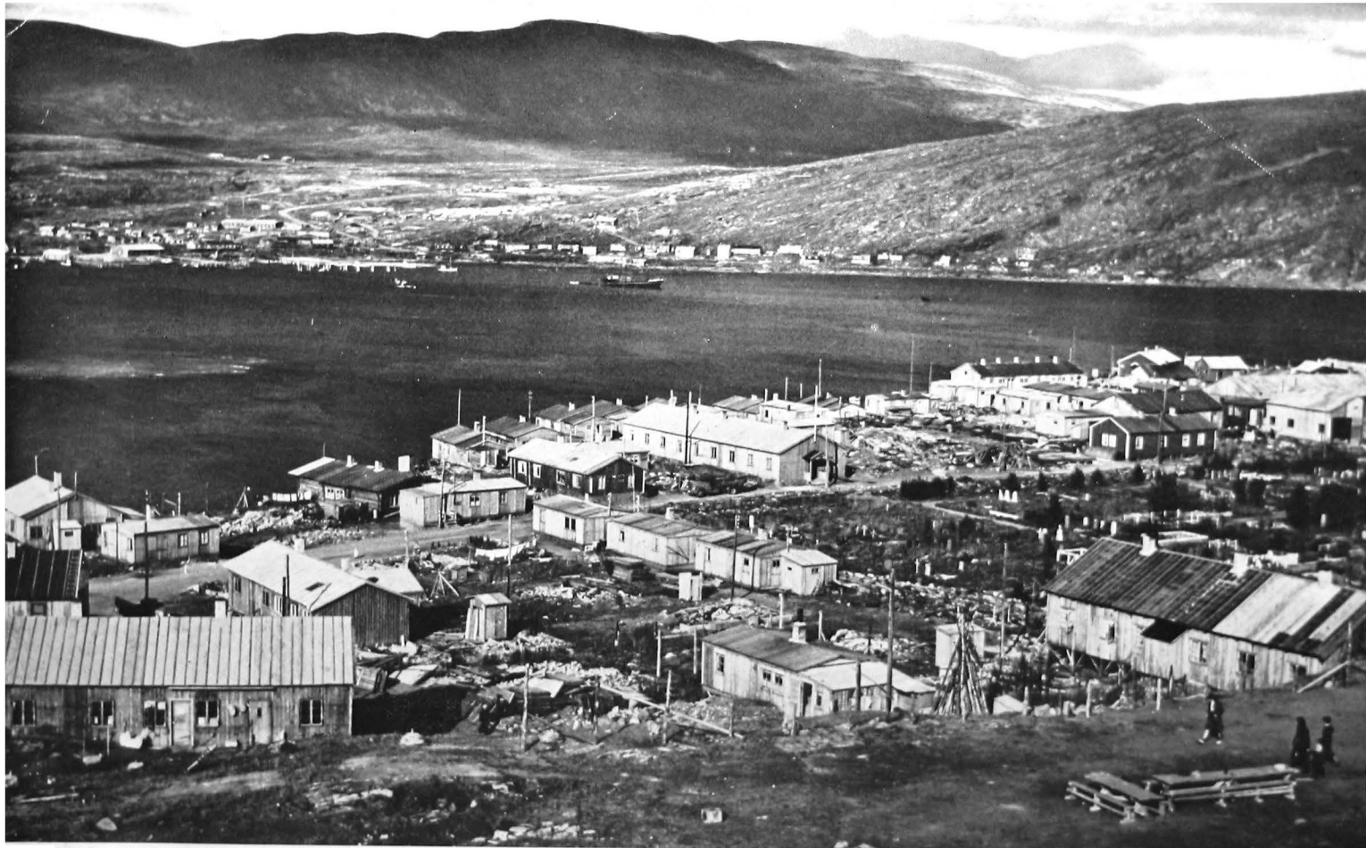
War-devastated Hammerfest under reconstruction.
