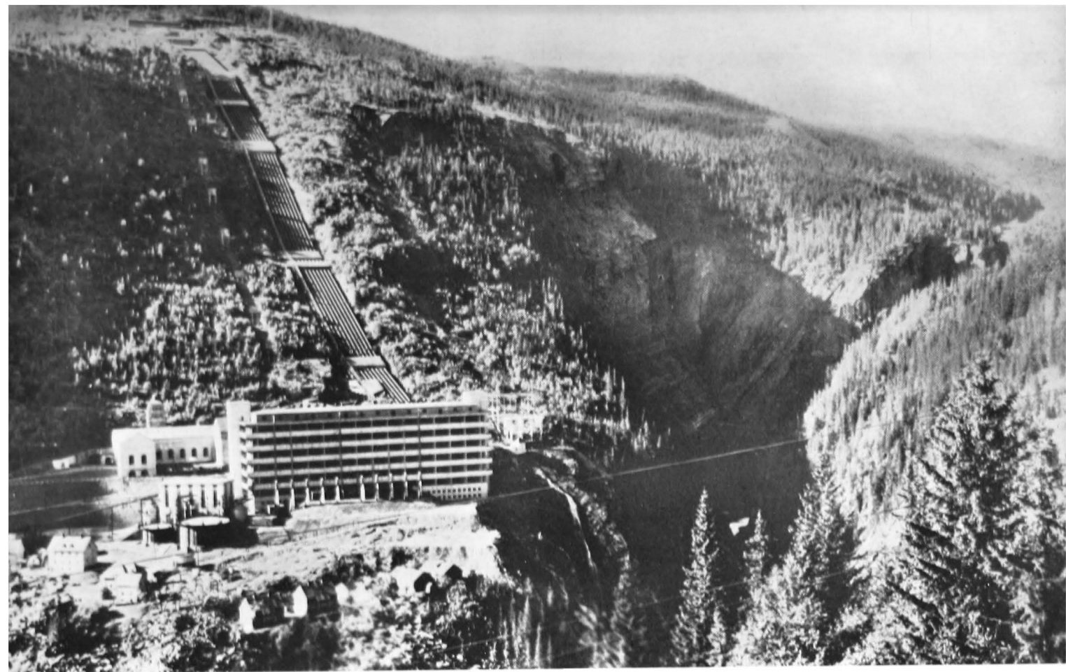
Power Station, Rjukan.
