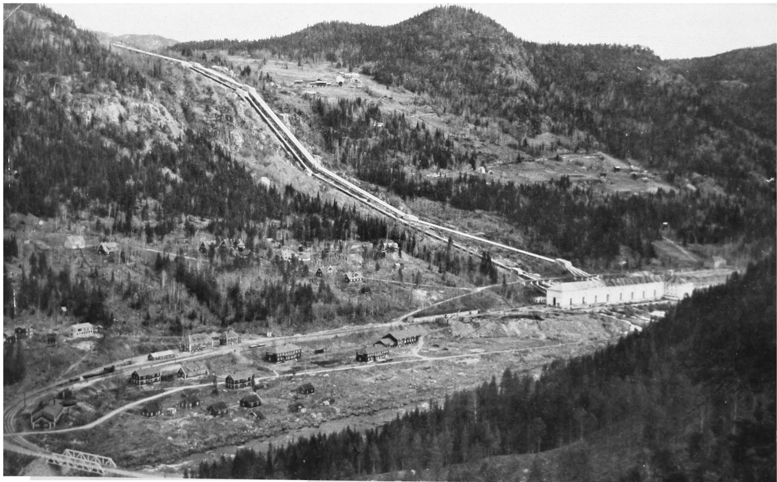
Hydro electric plant, Nore. Official photo.
