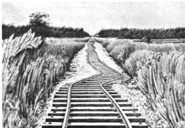
Fig. 25. Railway line in North Bengal after the earthquake of 1897
