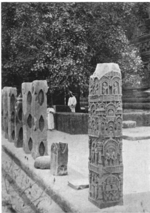
Fig. 37. Railing and sacred tree at Bodhi Gaya
