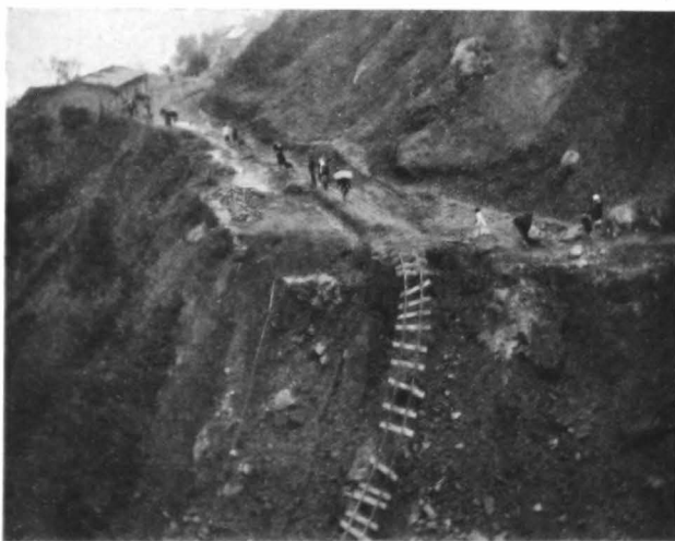
Fig. 20. Landslip on the Darjeeling Railway, 1899
