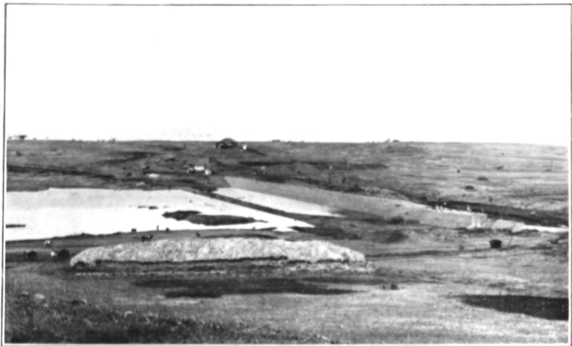
His Highness Shri RAJARAM CHHATRAPATI Tank ( under construction ).
