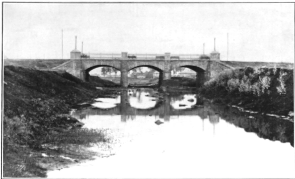
Lady Wilson Bridge.
