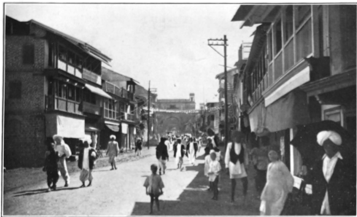
Bhavsingji Road (widened).
