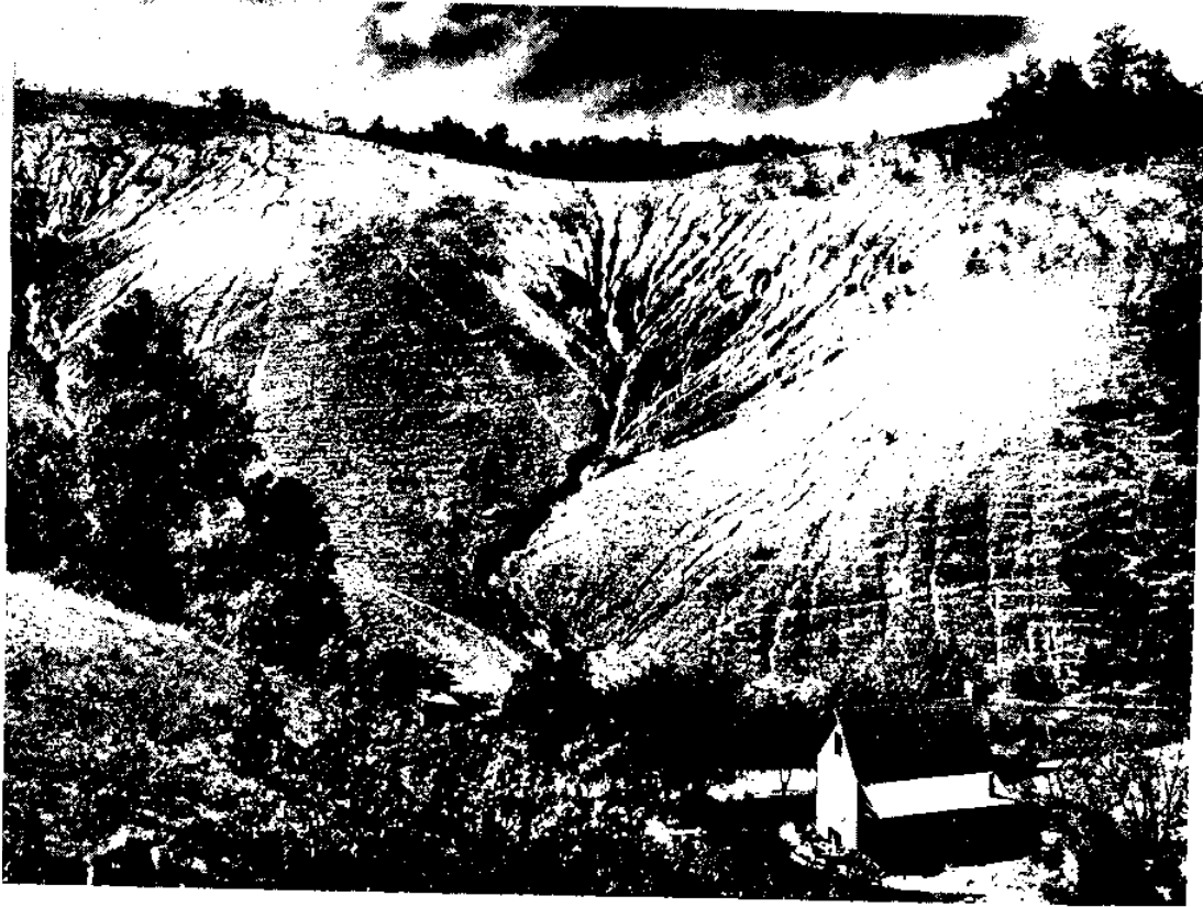
This is what 50 inches of rain a year does to a neglected slope.
